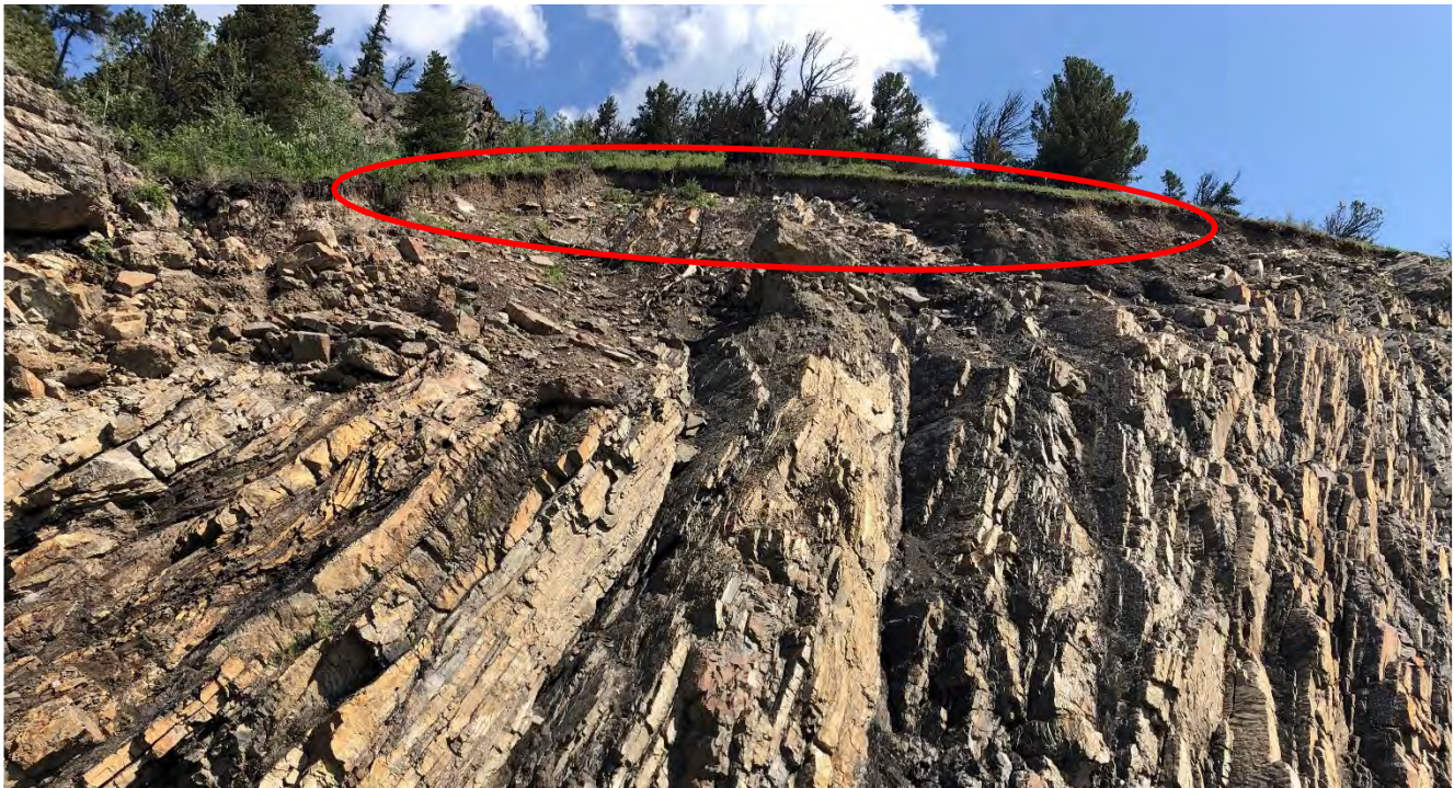
Photo 4 Erosion of soil at brow of slope leading to rockfalls and debris fans in the ditch.
