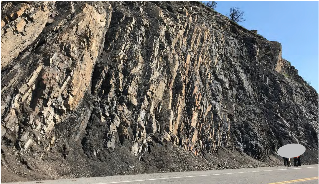
Photo 4 Erosion of soil at brow of slope leading to rockfalls and debris fans in the ditch.
