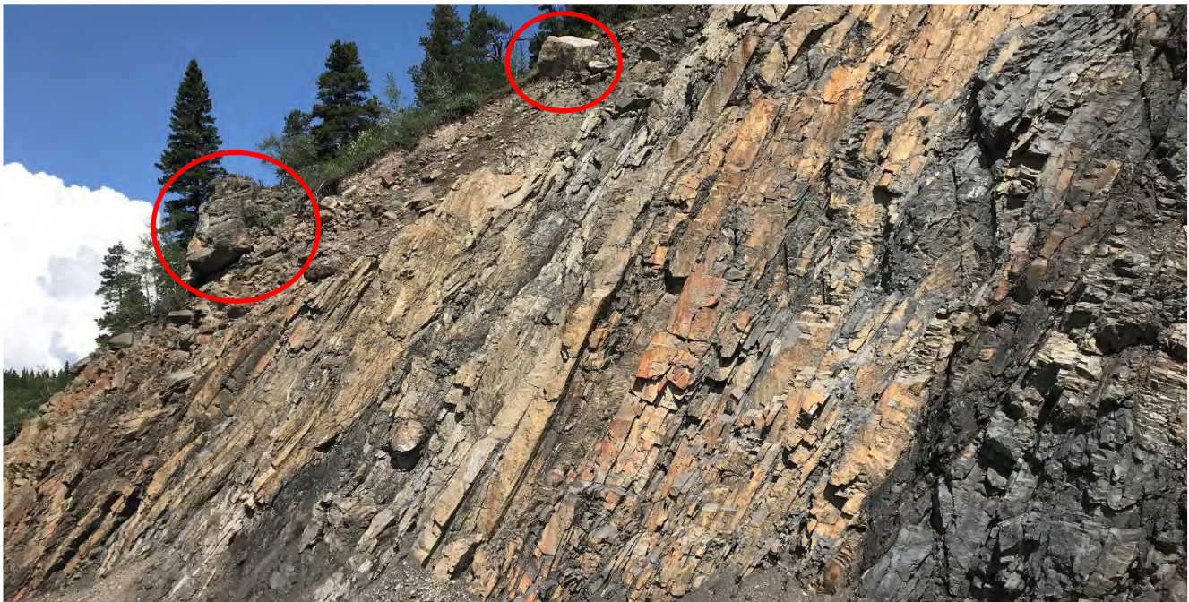
Photo 2 Loose blocks and boulders up to 0.5 m x 0.5 m x 0.5 m present along the length of the rock slope. Note large boulder at crest of slope. Photo was taken facing west on July 8, 2021.
