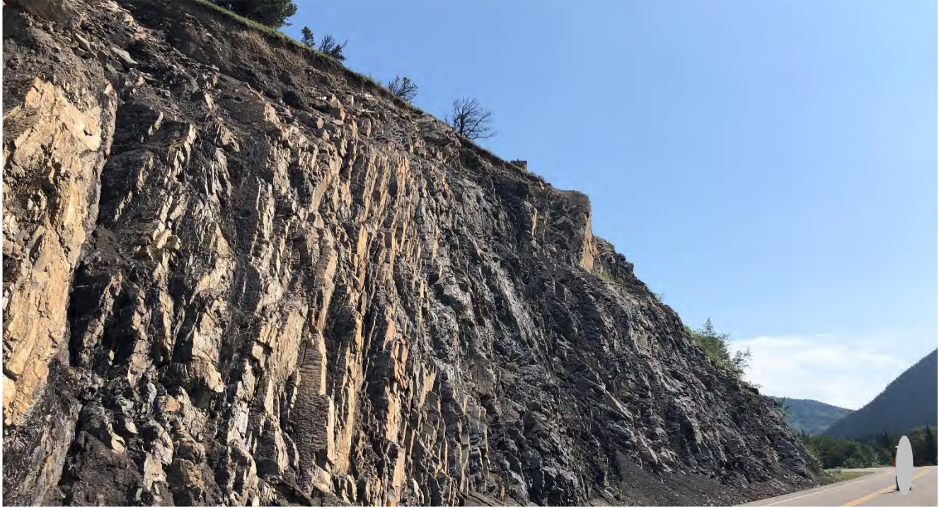
Photo 2 Loose blocks and boulders up to 0.5 m x 0.5 m x 0.5 m present along the length of the rock slope. Note large boulder at crest of slope. Photo was taken facing west on July 8, 2021.
