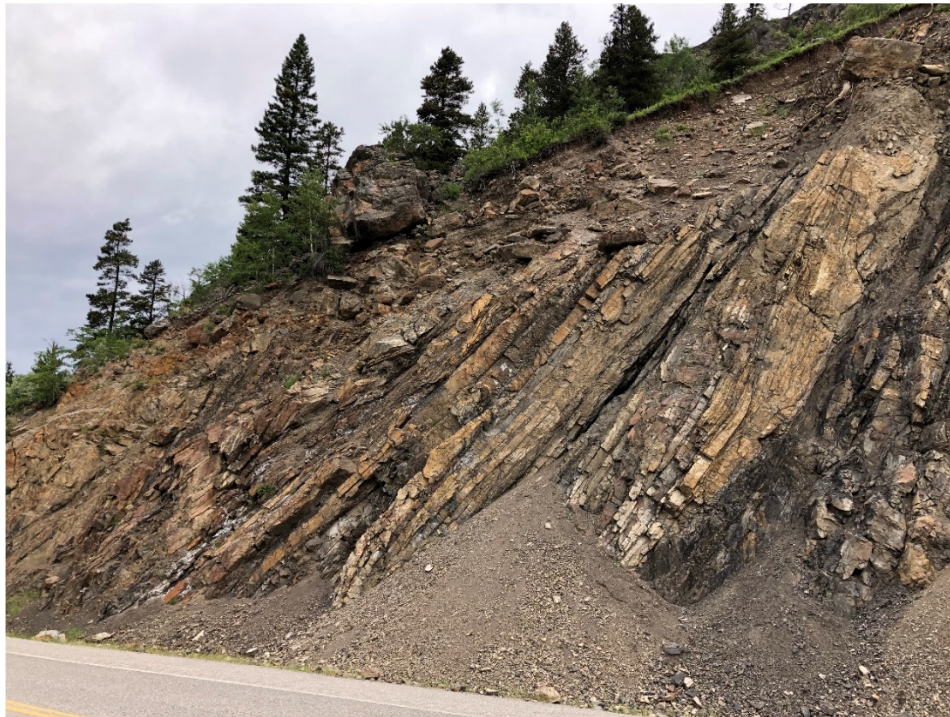
Photo 4 Erosion of soil at brow of slope, leading to rockfalls and debris fans in the ditch.
