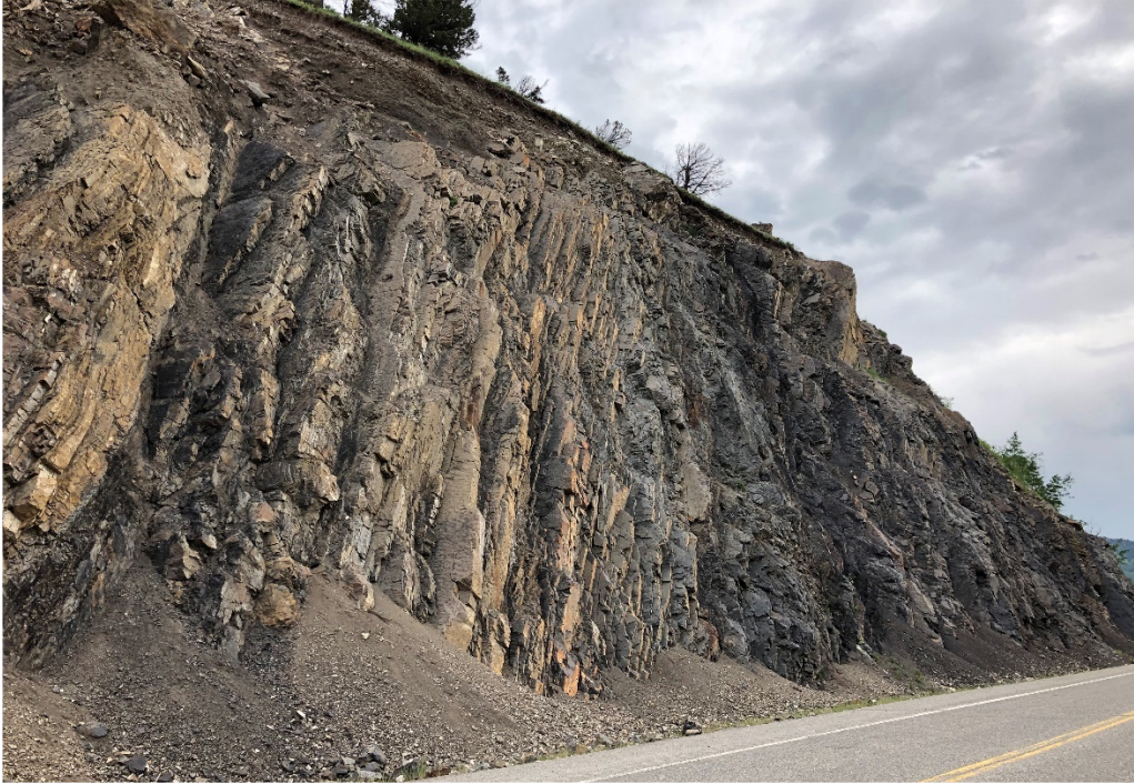
Photo 2 Loose blocks and boulders up to 0.5 m x 0.5 m x 0.5 m present along the length of the rock slope. Note large boulder at crest of slope. Photo was taken facing west on July 7, 2020.
