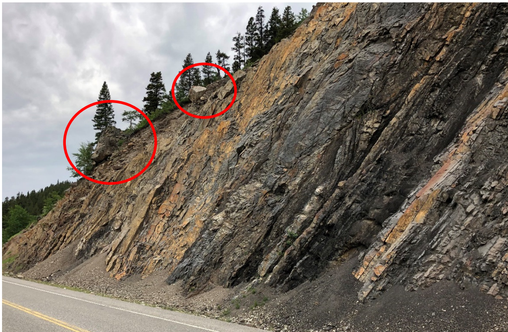
Photo 2 Loose blocks and boulders up to 0.5 m x 0.5 m x 0.5 m present along the length of the rock slope. Note large boulder at crest of slope. Photo was taken facing west on July 7, 2020.
