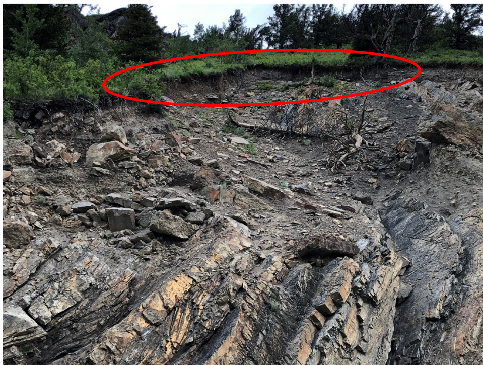
Photo 4 Erosion of soil at brow of slope, leading to rockfalls and debris fans in the ditch.
