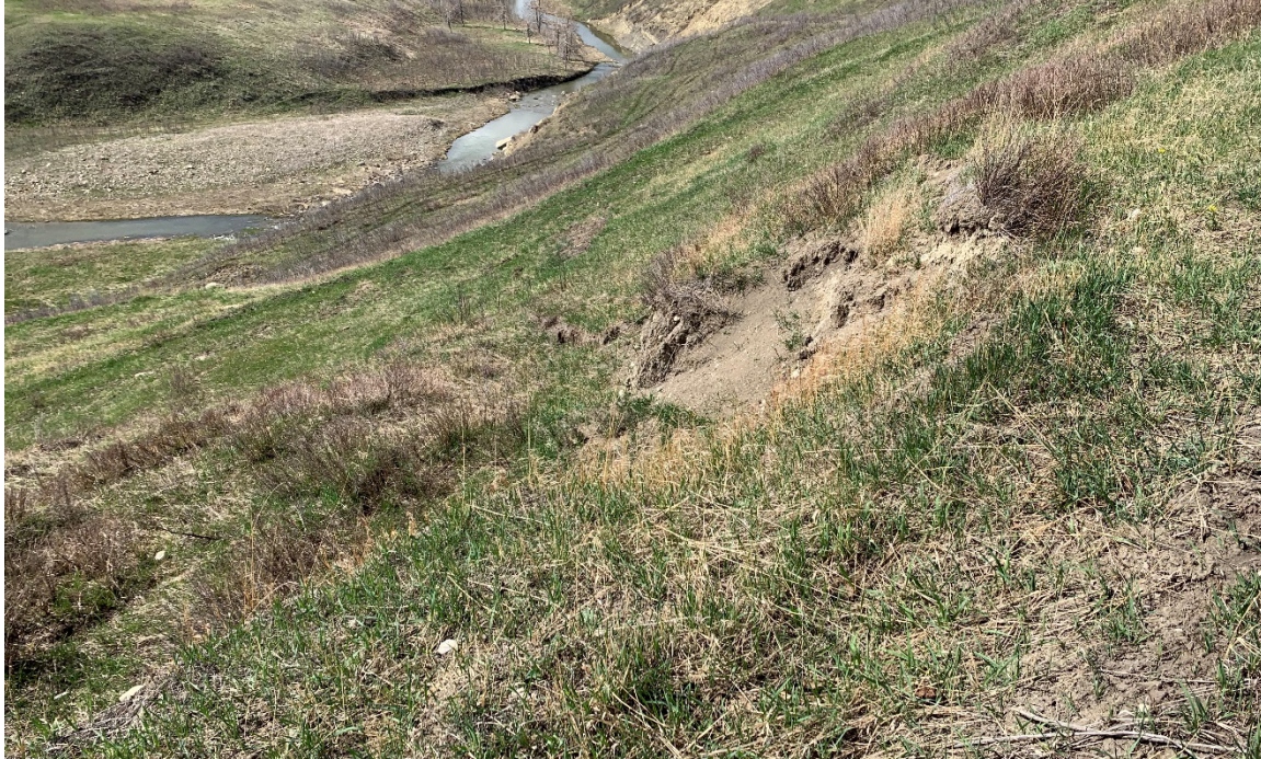
Photo 5 Site B slope. Photo was taken facing north on May 9, 2023.
