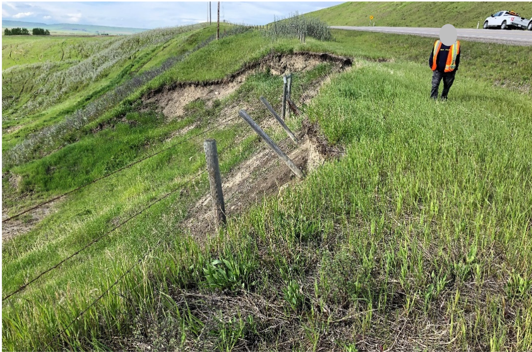
Photo 2 Site A: Instrumentation bench at mid slope of slide. Area around SI is wet. Photo was taken facing west on June 8, 2020.
