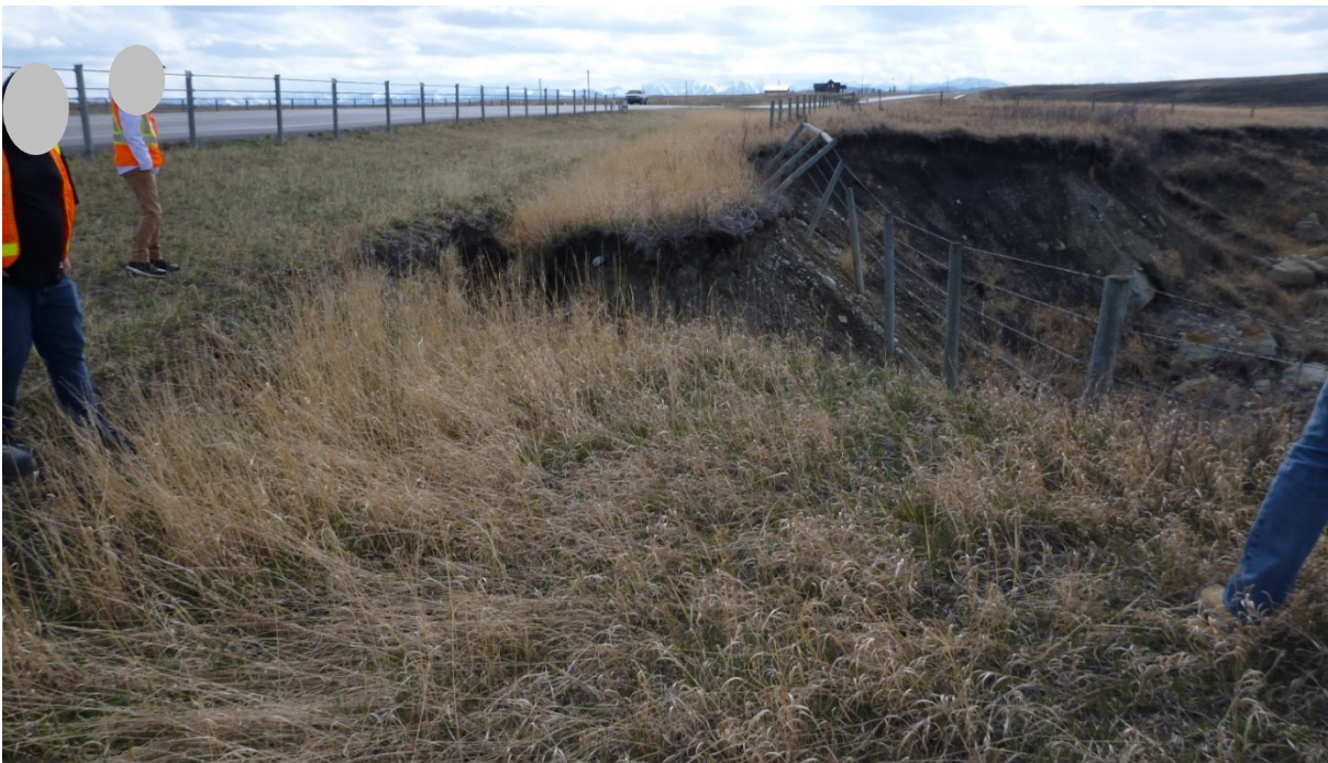
Photo 6 Site C: Creek erosion failure extending into highway ditch. Utility cable hanging across failure. Photo was taken facing southwest on May 6, 2019.
