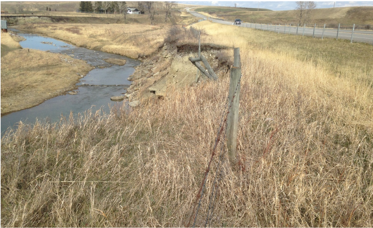
Photo 6 Site C: Creek erosion failure extending into highway ditch. Utility cable hanging across failure. Photo was taken facing southwest on May 6, 2019.
