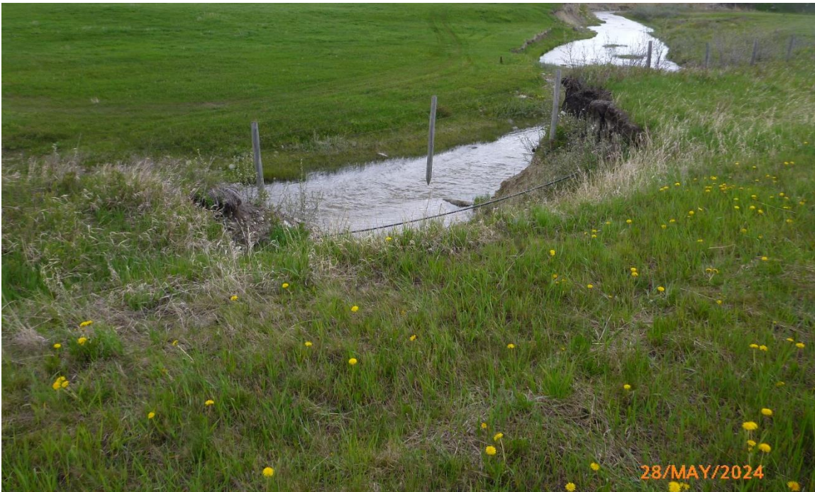
Photo 2 Bank erosion on the outside of a sharp meander bend. Fence line undermined. Utility cable exposed. Photo was taken facing west on May 28, 2024.
