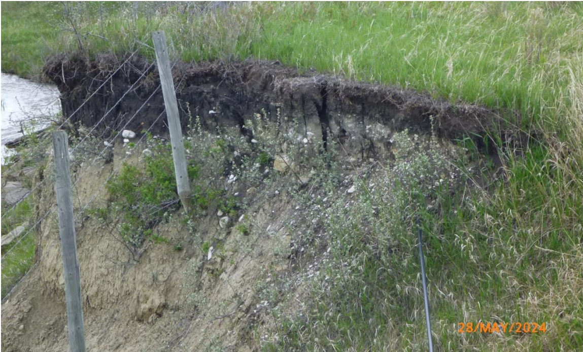
Photo 2 Bank erosion on the outside of a sharp meander bend. Fence line undermined. Utility cable exposed. Photo was taken facing west on May 28, 2024.
