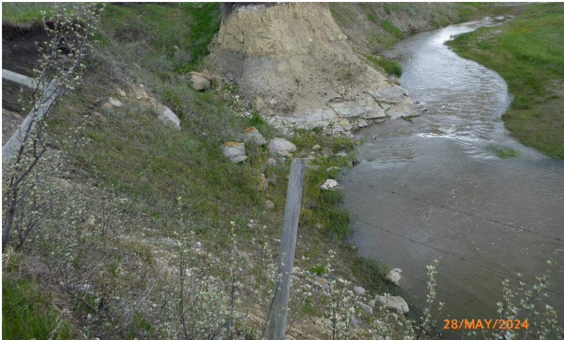
Photo 4 View of erosion north of fence undermining. Ditch flows discharge into erosion area. Photo was taken facing north on May 28, 2024.
