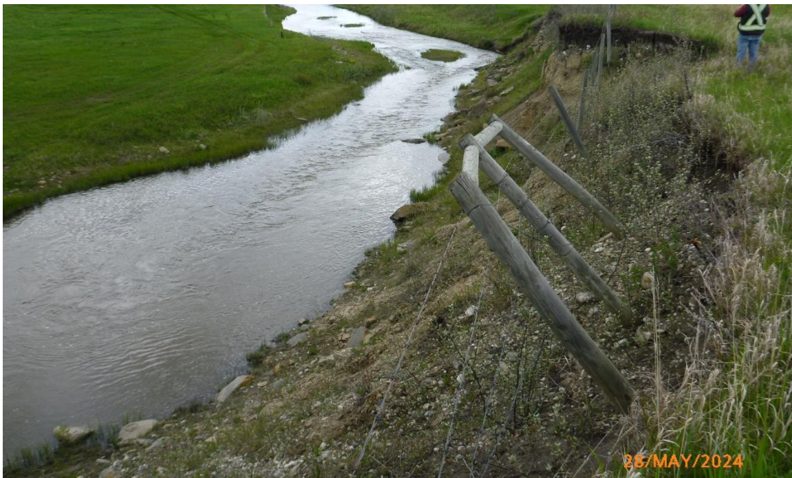
Photo 4 View of erosion north of fence undermining. Ditch flows discharge into erosion area. Photo was taken facing north on May 28, 2024.
