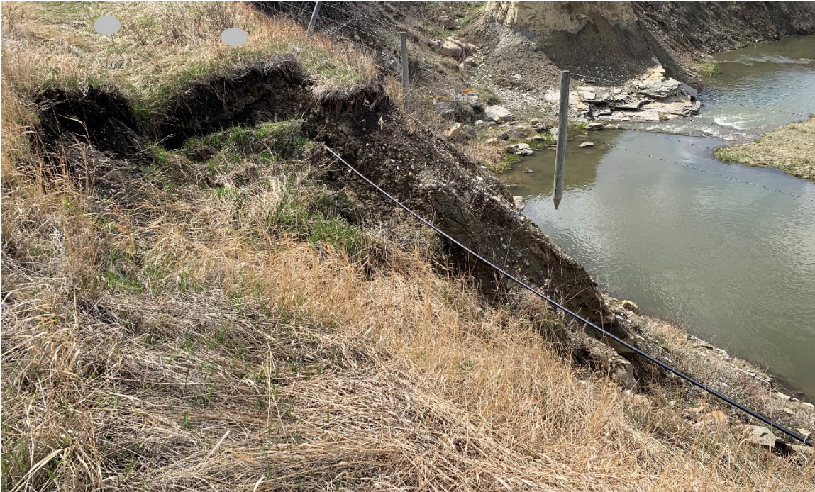
Photo 2 Bank erosion on the outside of a sharp meander bend. Fence line undermined. Utility cable exposed. Photo was taken facing west on May 9, 2023.
