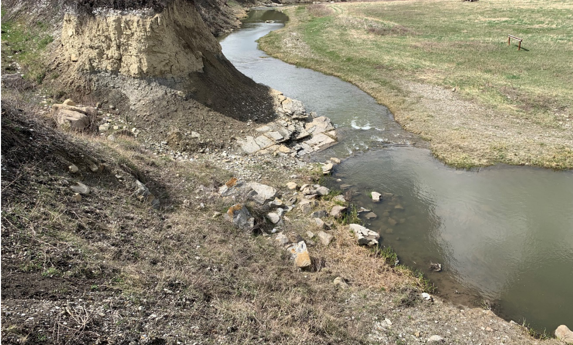
Photo 5 Erosion feature. Photo was taken facing southwest on May 9, 2023.
