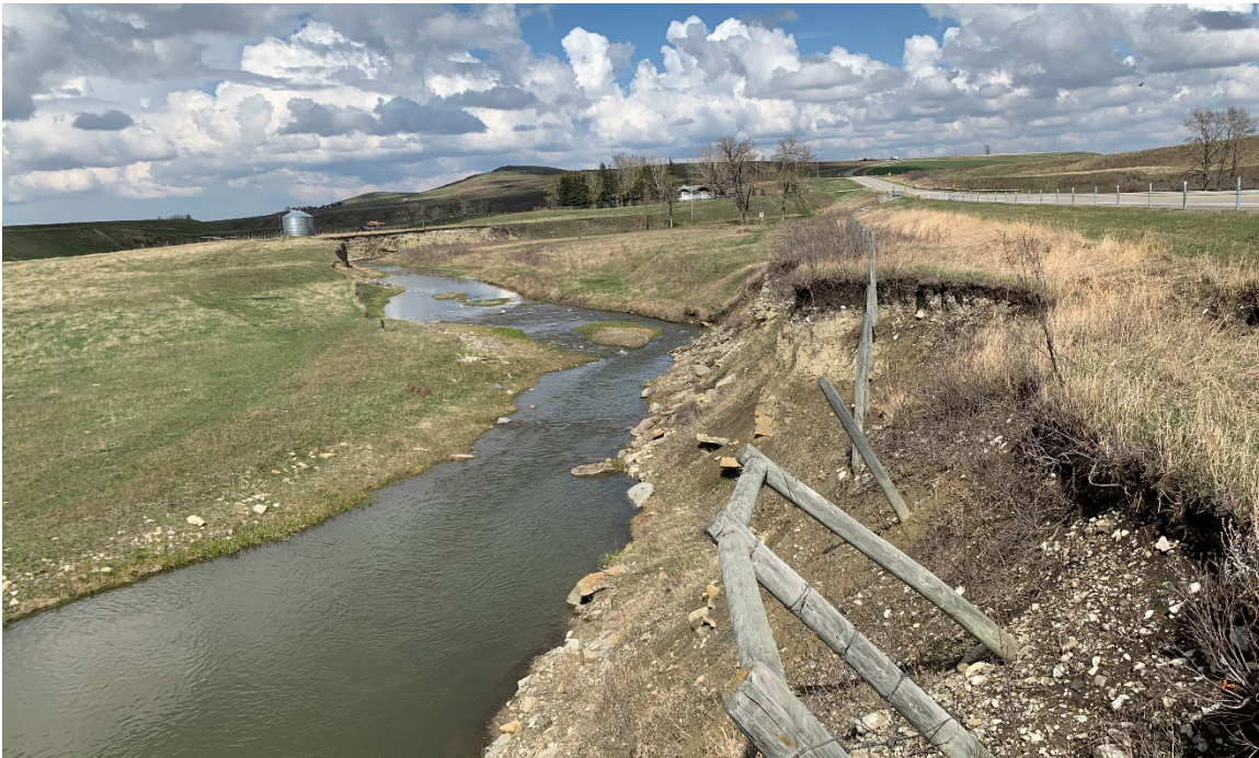
Photo 4 View of erosion north of fence undermining. Ditch flows discharge into erosion area. Photo was taken facing north on May 9, 2023.
