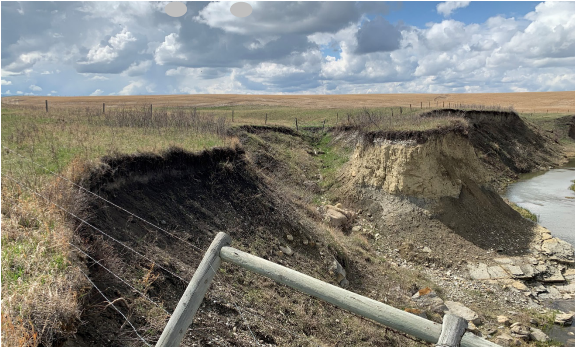
Photo 4 View of erosion north of fence undermining. Ditch flows discharge into erosion area. Photo was taken facing north on May 9, 2023.
