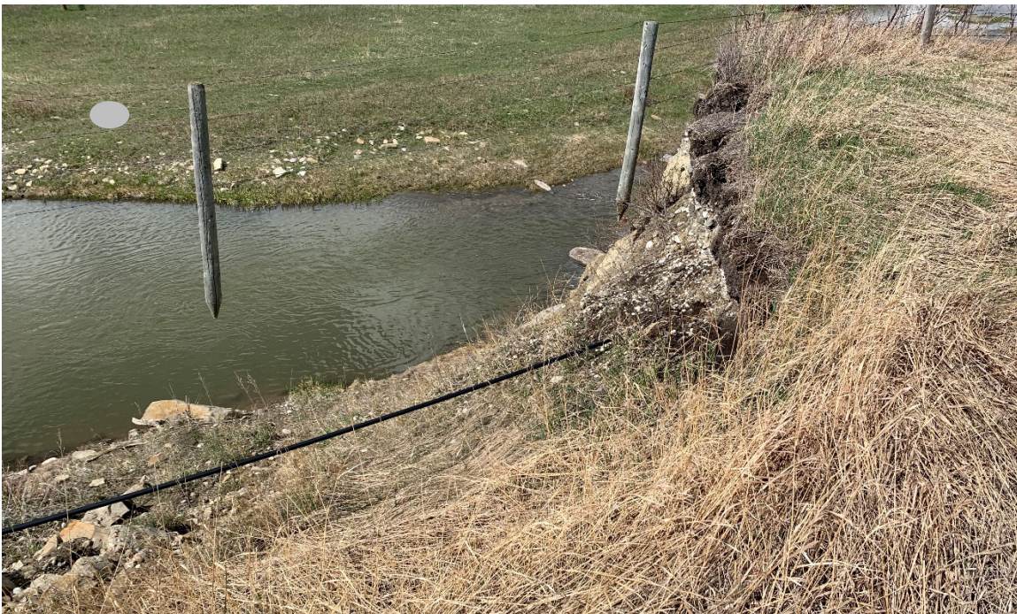
Photo 2 Bank erosion on the outside of a sharp meander bend. Fence line undermined. Utility cable exposed. Photo was taken facing west on May 9, 2023.
