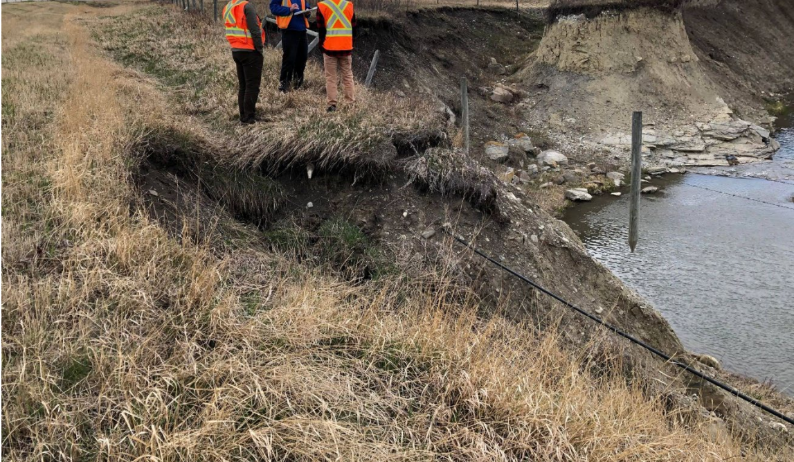
Photo 4 Tension cracking (indicated by red dashed line) near the fence and west end of the site. Photo taken May 16, 2022, facing northeast.
