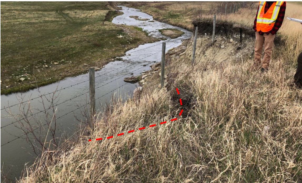
Photo 4 Tension cracking (indicated by red dashed line) near the fence and west end of the site. Photo taken May 16, 2022, facing northeast.
