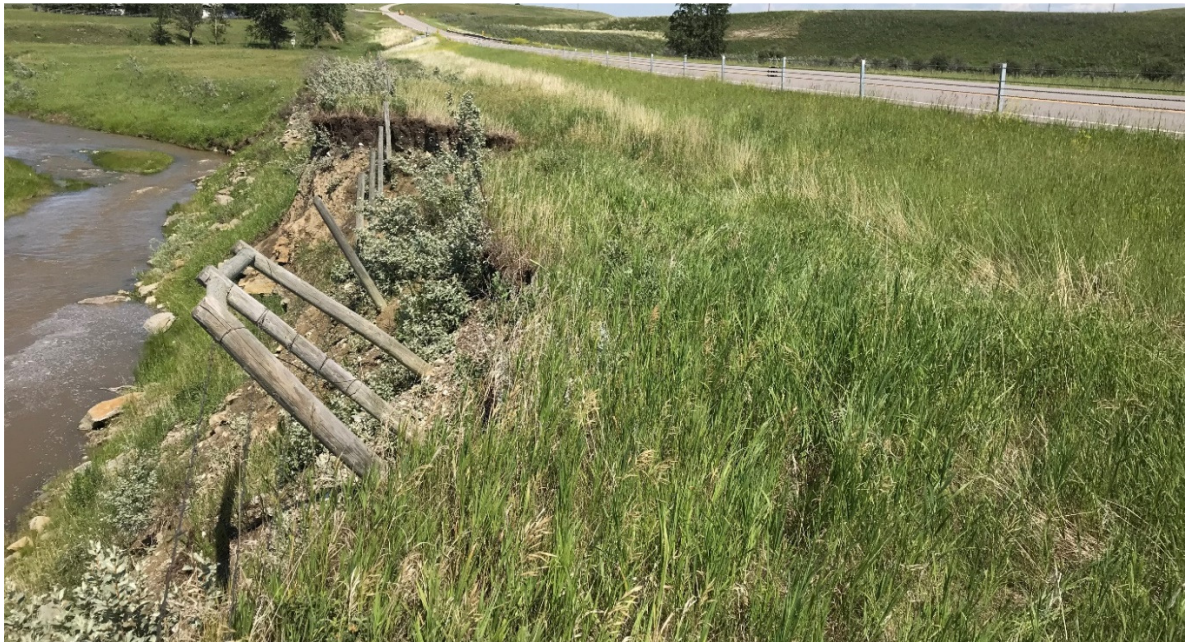
Photo 4 Tension cracking (red line) in highway right-of-way on the west flank of the erosion feature. Photo was taken facing northeast on July 9, 2021.
