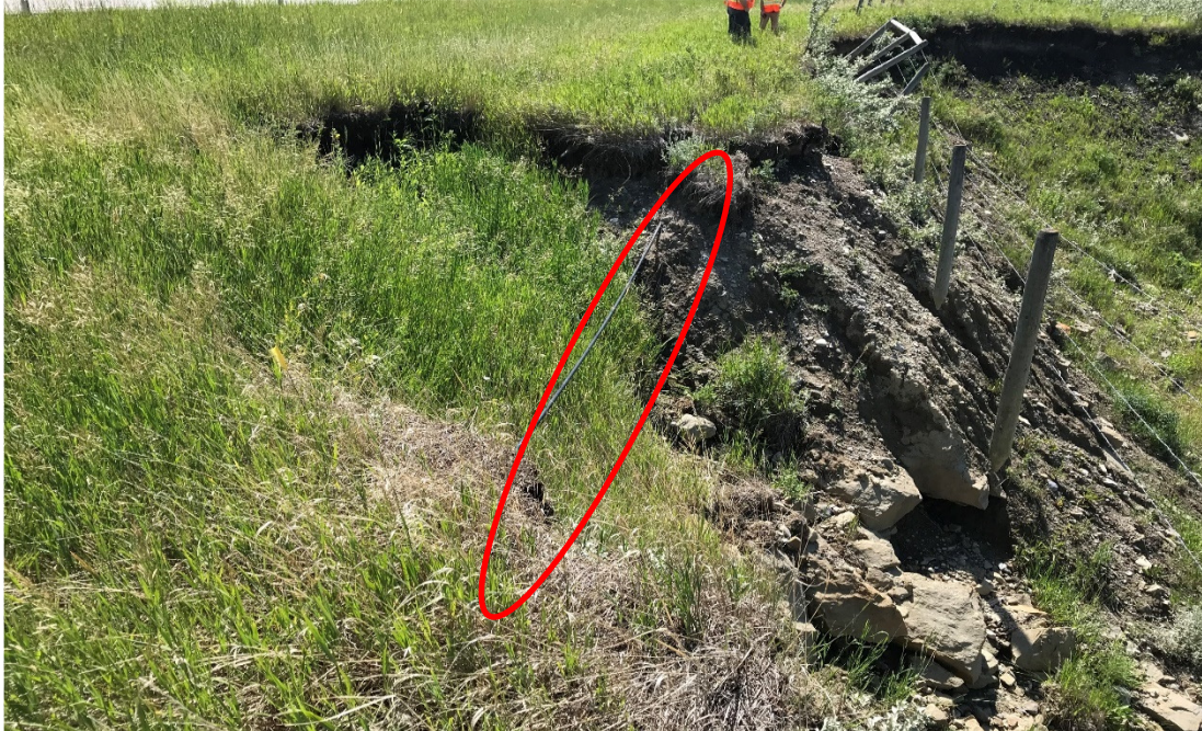
Photo 2 Bank erosion on the outside of a sharp meander bend. Fence line undermined. Photo was taken facing southwest on July 9, 2021.
