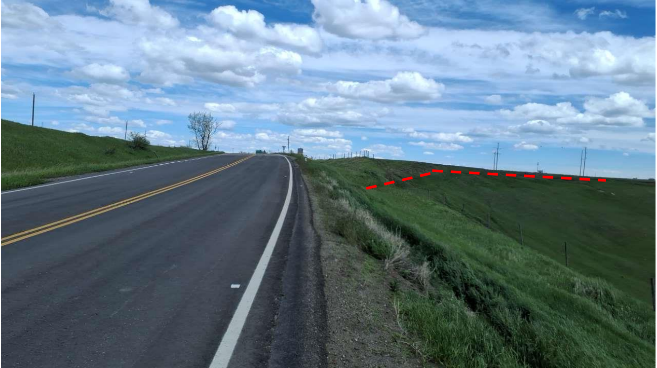
Photo 3 Head scarp of slide on coulee slope south of highway. Photo was taken May 19, 2022, facing east.
