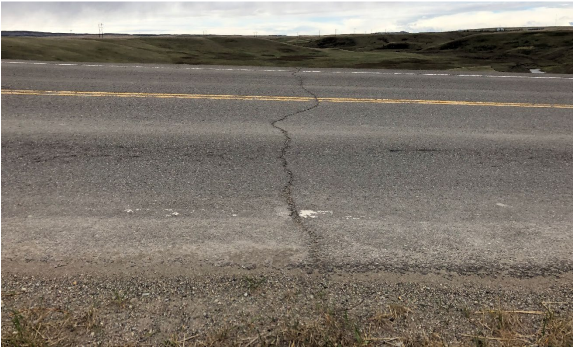
Photo 4 Head scarp of slide on coulee slope south of highway. Photo was taken May 19, 2022, facing southeast.
