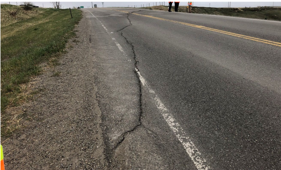
Photo 2 Pavement patching and milling due to ongoing slope movement. Cracking has extended through the overlay. Photo taken May 19, 2022, facing east.
