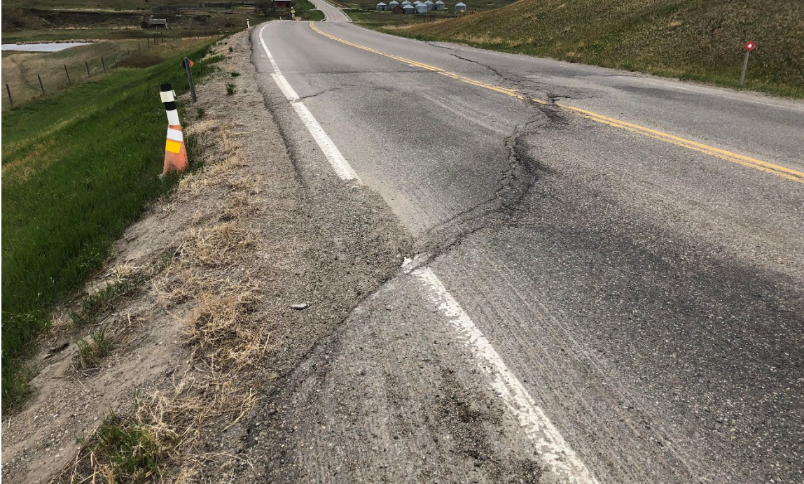
Photo 2 Pavement patching and milling due to ongoing slope movement. Cracking has extended through the overlay. Photo taken May 19, 2022, facing east.
