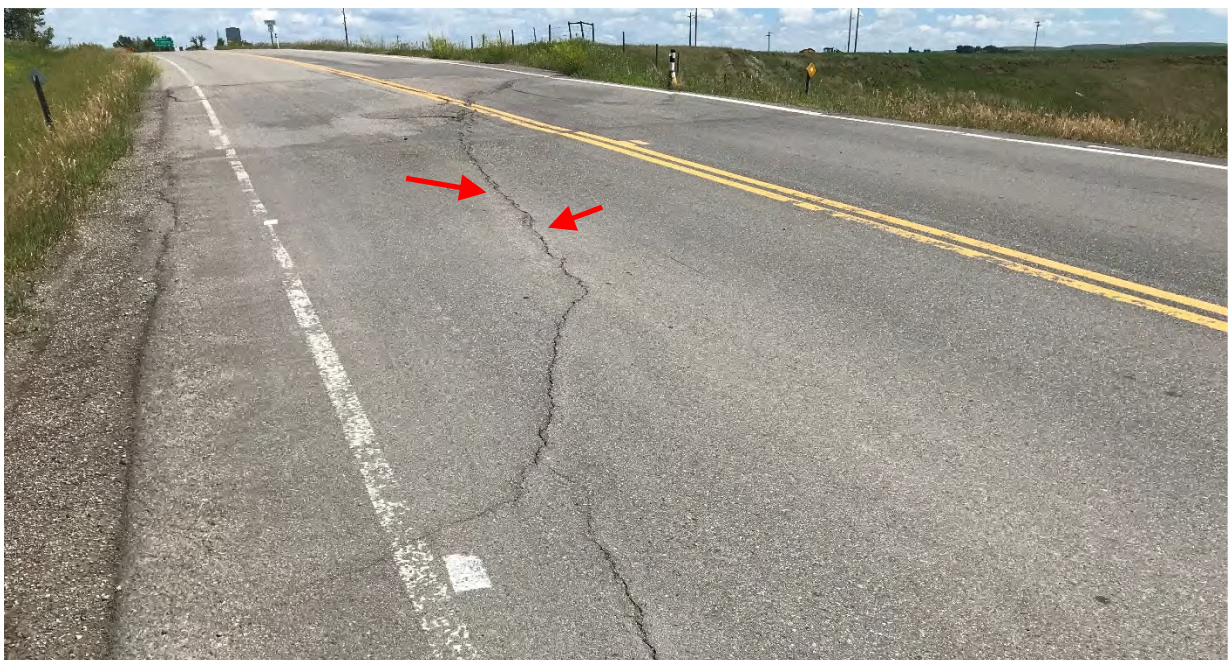
Photo 2 Pavement patching and milling due to ongoing slope movement. Cracking has extended through the recent overlay. Photo taken facing east on July 8, 2021.
