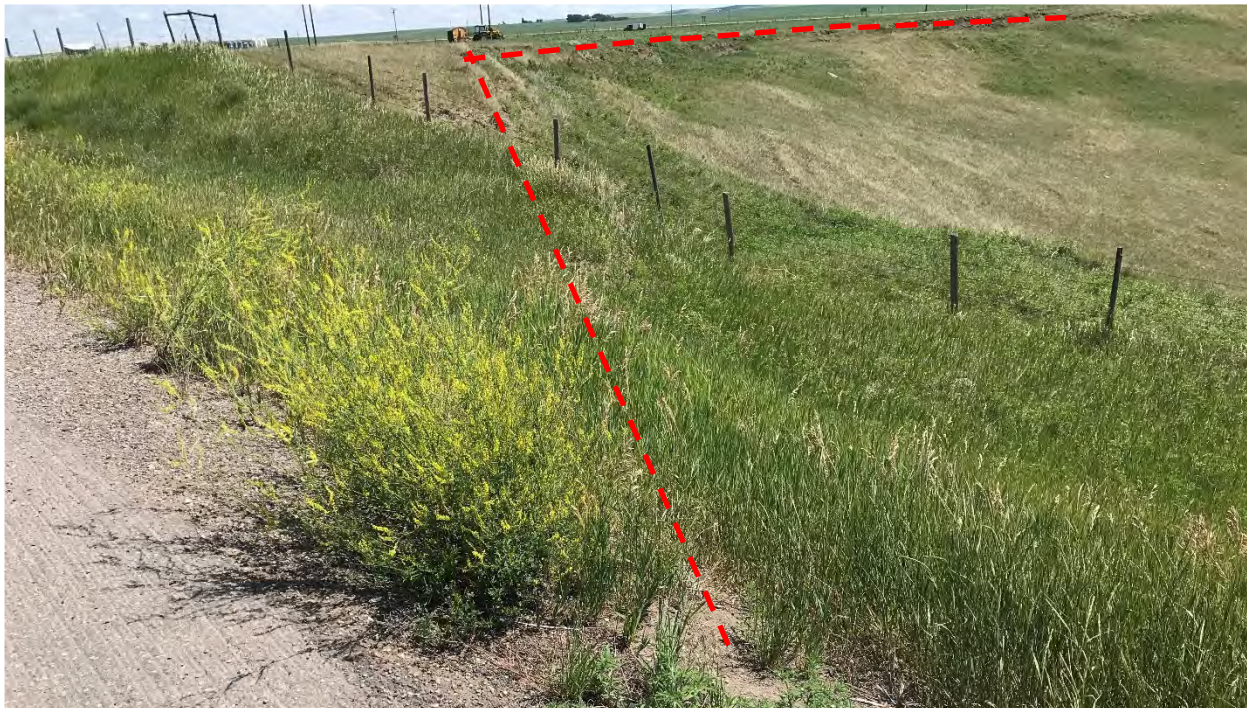
Photo 4 Head scarp of slide on coulee slope south of highway. Photo was taken facing southeast on July 8, 2021.
