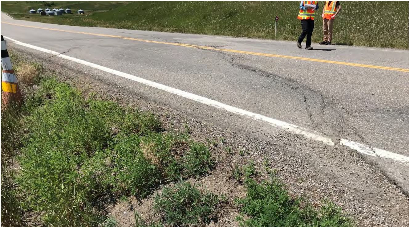
Photo 2 Pavement patching and milling due to ongoing slope movement. Cracking has extended through the recent overlay. Photo taken facing east on July 8, 2021.
