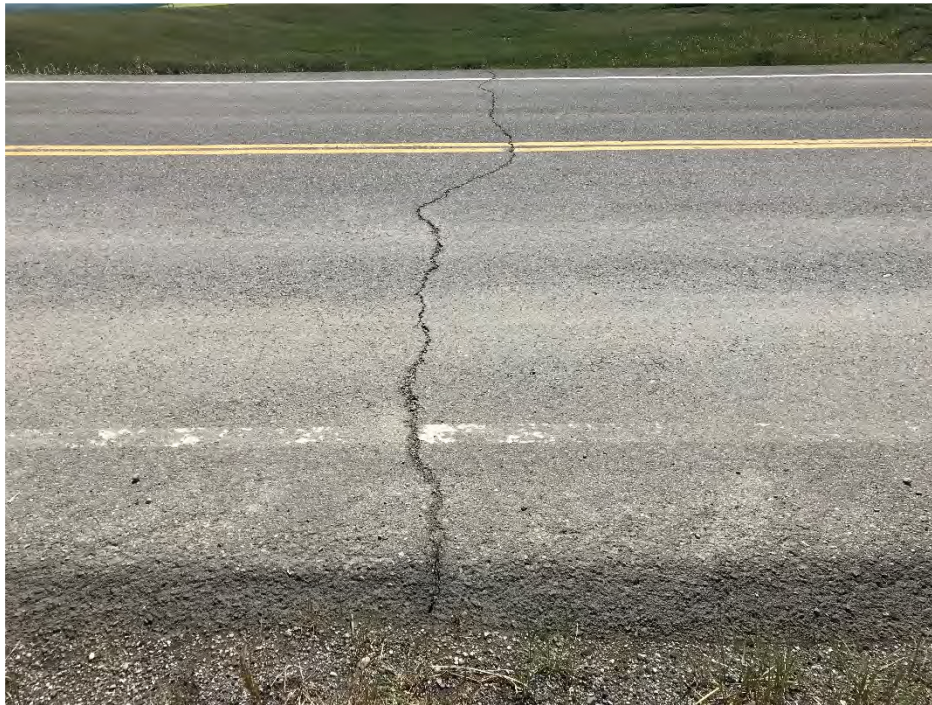
Photo 4 Head scarp of slide on coulee slope south of highway. Photo was taken facing southeast on July 8, 2021.
