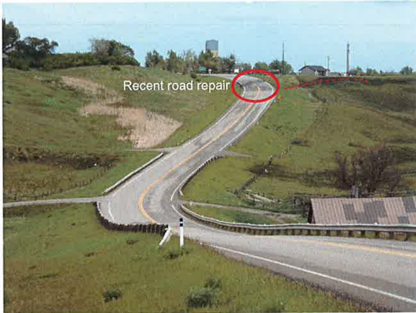
Photo 1 - (May 2015) – Site overview. Facing east towards site. Main headscarp marked with red dashed line.
