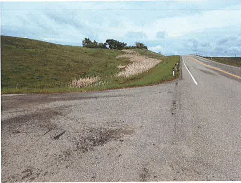
Photo 3 - (May 2015) – Facing east towards area of moist ground on north shoulder of Highway 505 indicated by cat tail vegetation.
