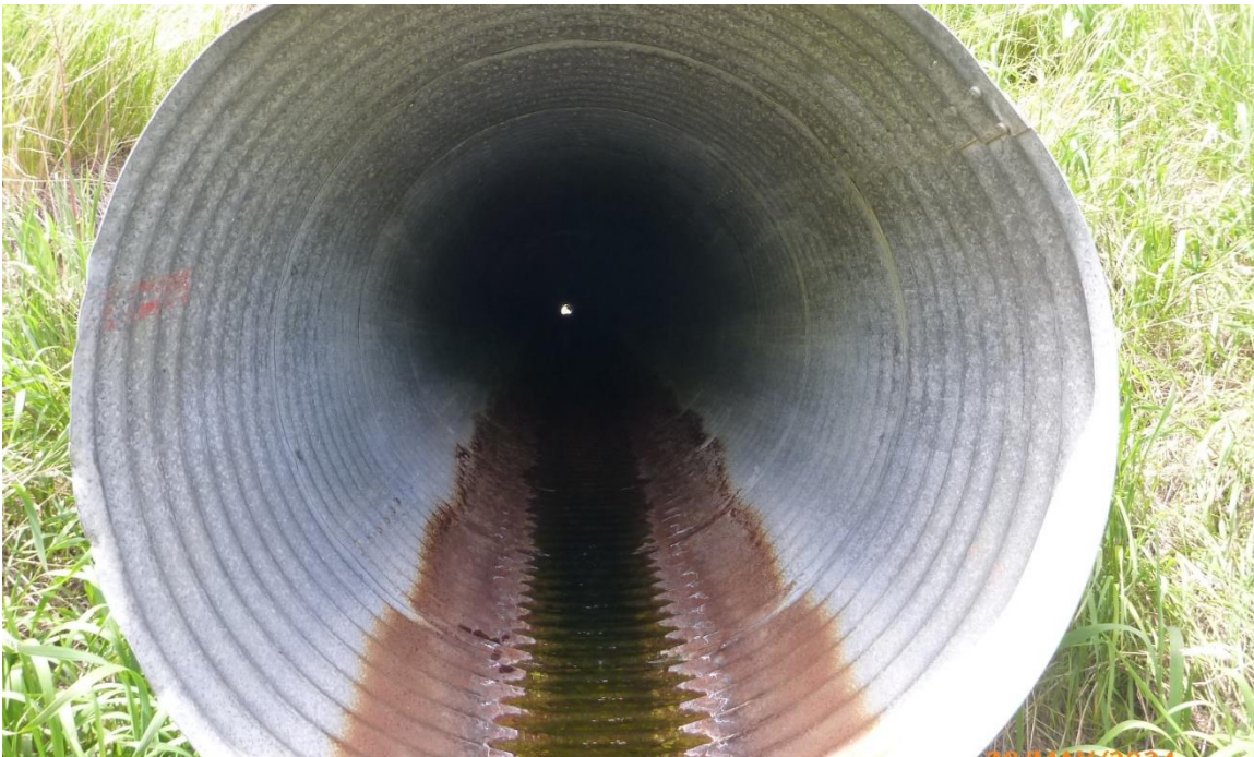
Photo 5 CSP culvert outlet near the left flank of the slide zone. The CSP culvert appears to be in good condition. Photo taken May 29, 2024, facing northwest.
