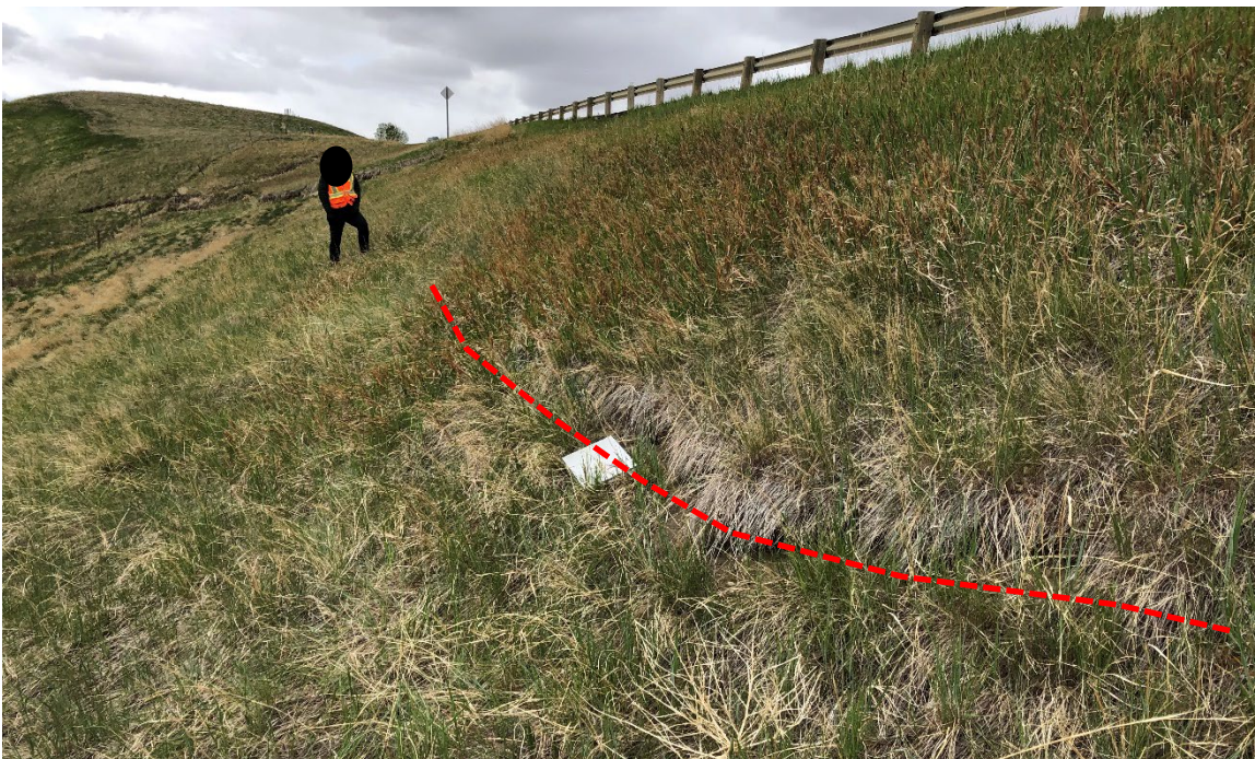
Photo 5 Tension crack on embankment fill (indicated by red dashed line) (WP 106) approximately 2 m below pavement elevation. Photo taken May 19, 2022, facing southwest.
