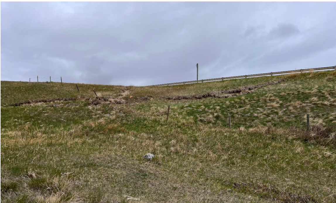
Photo 3 Head scarp on right flank. Photo taken on May 19, 2022, facing northwest.
