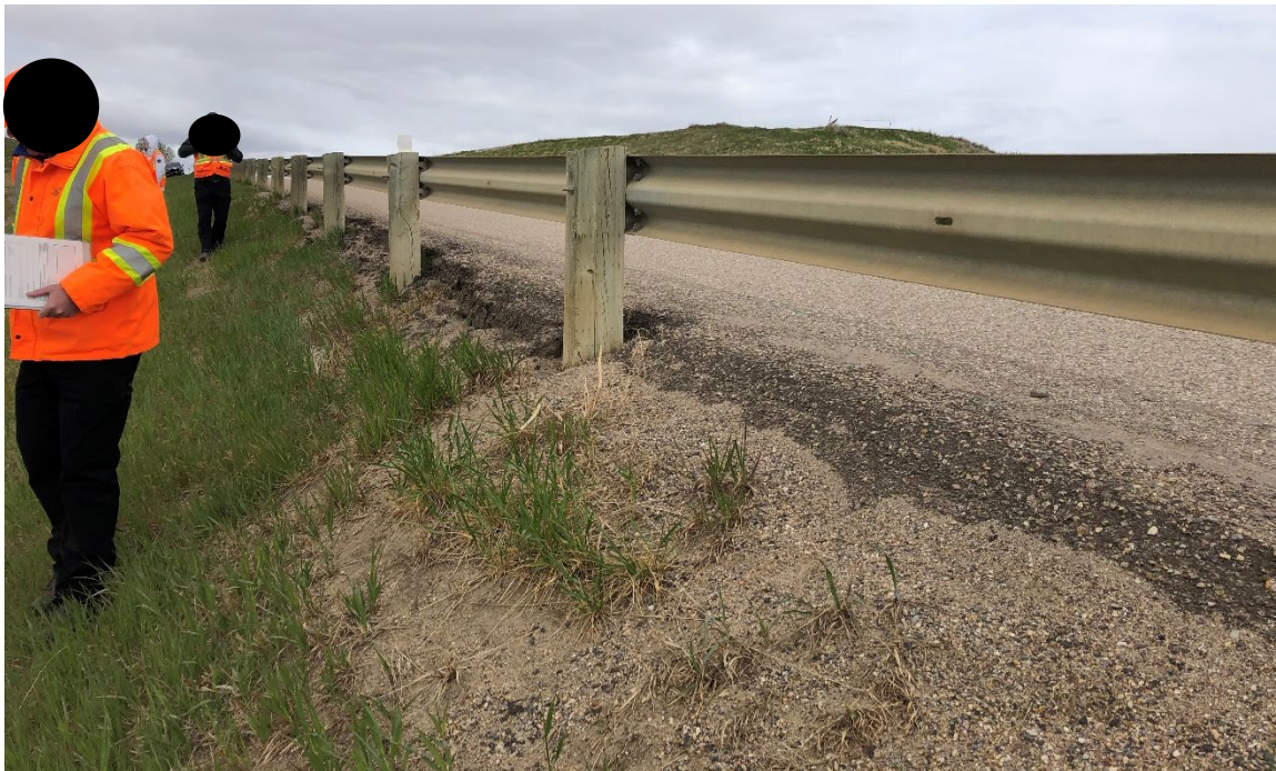
Photo 7 The head scarp at the edge of the pavement and is reducing the pavement support over approximately 18 m. Photo taken May 19, 2022, facing west.
