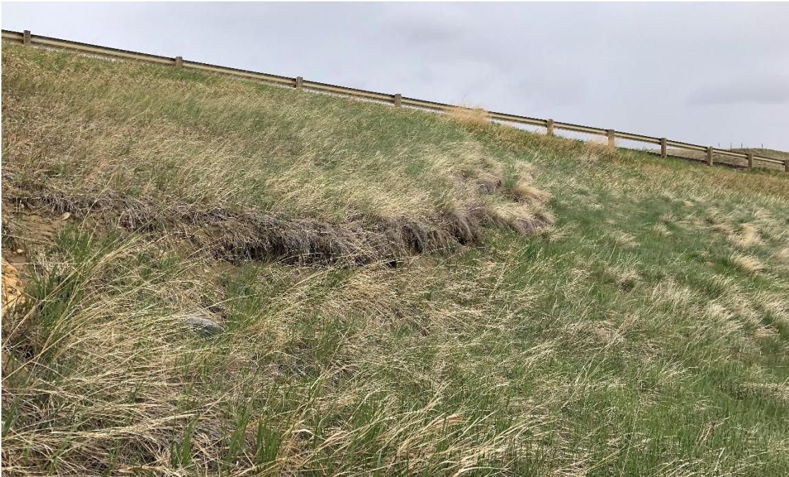
Photo 5 Tension crack on embankment fill (indicated by red dashed line) (WP 106) approximately 2 m below pavement elevation. Photo taken May 19, 2022, facing southwest.
