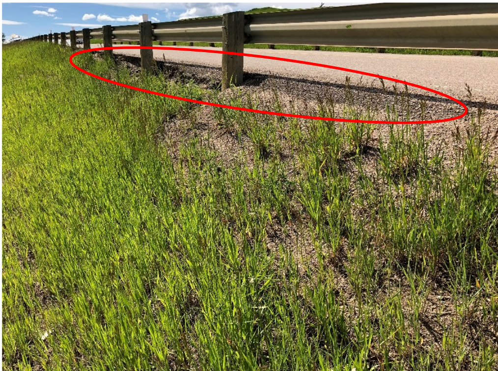
Photo 3 Head scarp at the edge of the pavement. Loss of pavement support over approximately 18 m length. Photo taken facing east on June 9, 2020.
