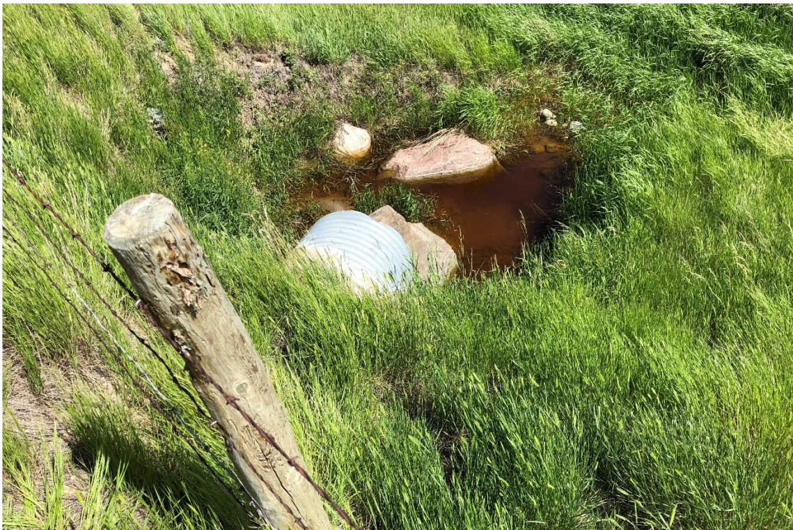
Photo 5 Culvert under the highway embankment on left flank of slide zone. Photo taken facing south on June 9, 2020.
