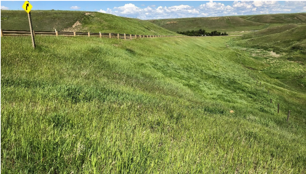
Photo 3 Head scarp at the edge of the pavement. Loss of pavement support over approximately 18 m length. Photo taken facing east on June 9, 2020.
