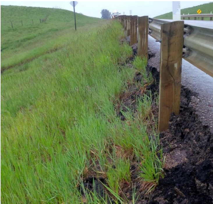
Photo 3 Head scarp right at edge of pavement. Loss of pavement ~ 15 m length and guardrail was pulled into lane by maintenance. Photo towards west on June 16, 2016.
