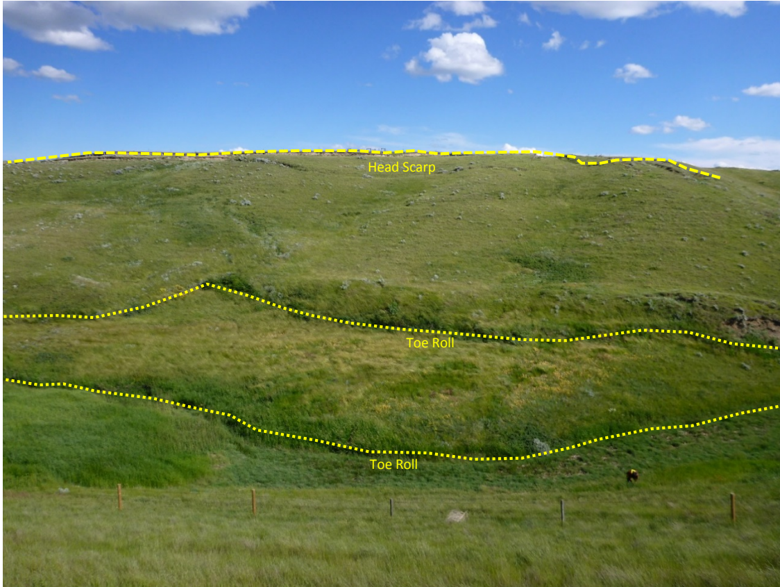
Photo 4 Large translational landslide on north facing slope south of the subject site. The supports the hypothesis that a horizontal weak layer is controlling translational slide movement in the vicinity. Photo towards south on June 16, 2016.
