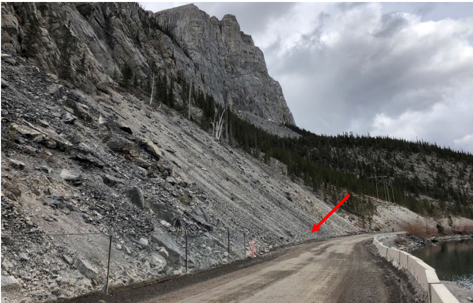
Photo 2 Location north of the highway where the installation of a wire mesh should be completed to mitigate the rockfall hazard (indicated by red arrow). Photo taken May 17, 2022, facing northeast.
