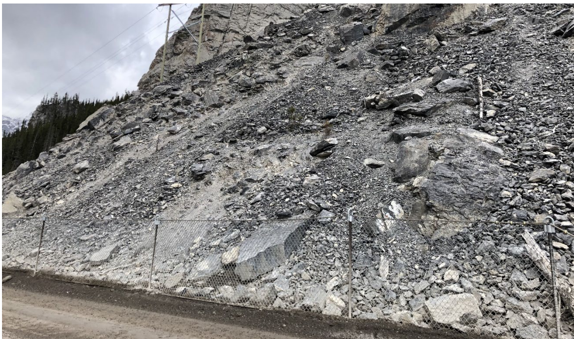
Photo 4 Rock slope north of the highway. Debris has accumulated behind the rock fence since and requires removal. No significant change since the 2021 inspection. Photo taken May 17, 2022, facing southwest.
