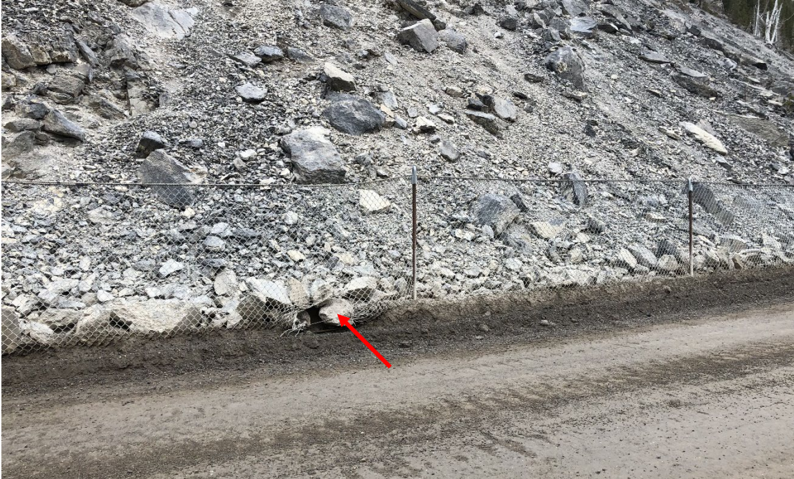
Photo 4 Rock slope north of the highway. Debris has accumulated behind the rock fence since and requires removal. No significant change since the 2021 inspection. Photo taken May 17, 2022, facing southwest.
