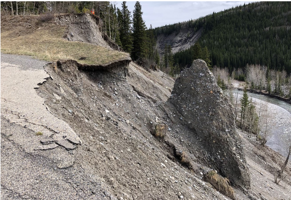
Photo 4 A large block has failed and dropped downslope (WP 87). The block does not appear to have changed significantly since the 2021 inspection. Photo taken May 16, 2022, facing east.
