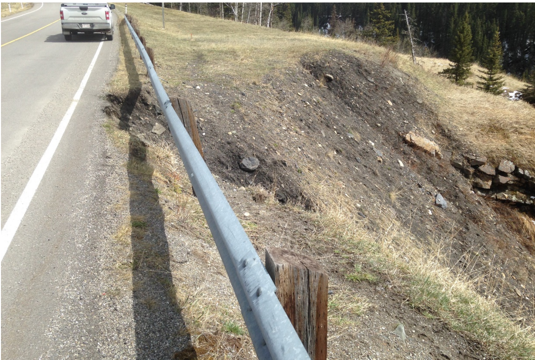
Photo 2 Ongoing slope retrogression impacting the highway. Photo was taken facing east on May 6, 2019.
