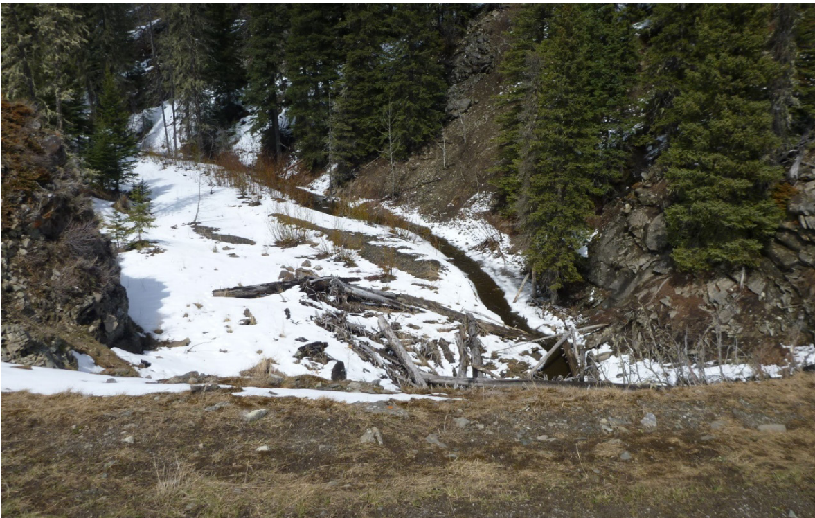
Photo 4 Debris and vegetation at upstream entrance to culvert. Photo was taken facing north on May 6, 2019.
