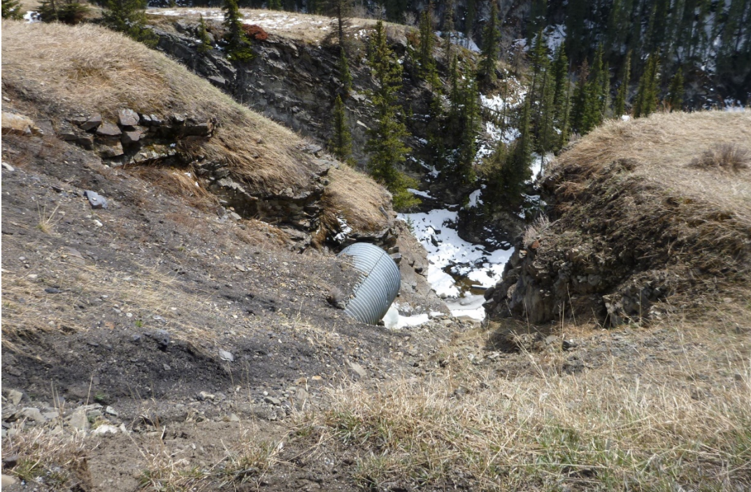
Photo 2 Ongoing slope retrogression impacting the highway. Photo was taken facing east on May 6, 2019.
