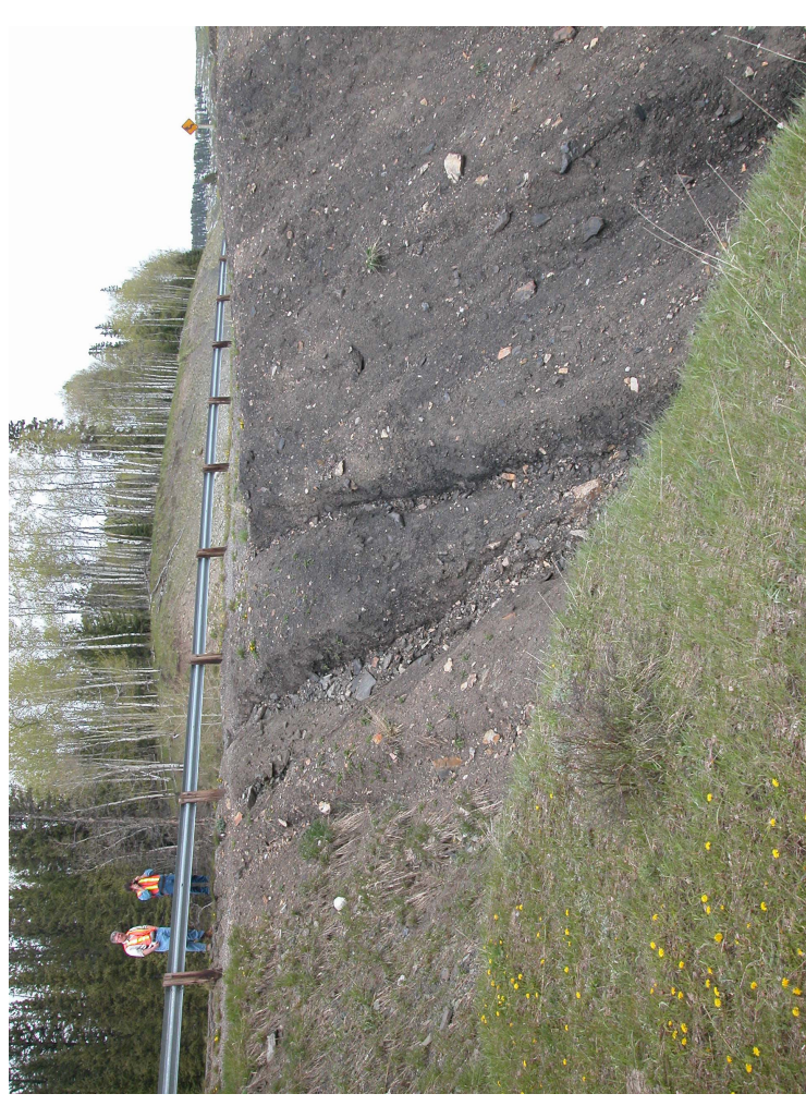
Photo S13-3 (lower left) – May 2004 – facing east across the site, showing the relative position of the gully erosion in the fill embankment slope face and the guardrail/road surface. Note the pile of rockfall debris that has been hauled from a site to the east and stockpiled here for later disposal into the gully downstream of the road.
