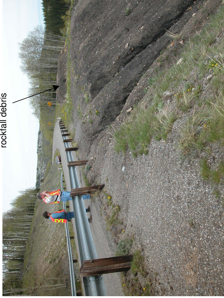
Photo S13-3 (lower left) – May 2004 – facing east across the site, showing the relative position of the gully erosion in the fill embankment slope face and the guardrail/road surface. Note the pile of rockfall debris that has been hauled from a site to the east and stockpiled here for later disposal into the gully downstream of the road.
