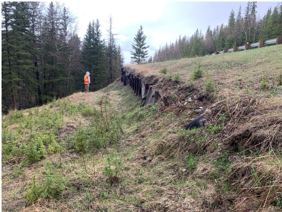
Photo 4 Site B: Pile wall is located downslope to the west of the highway. Soil movement downslope of the wall has exposed 2 to 3 m of steel pile over a length of approximately 30 m. Photo was taken facing north on May 11, 2023.
