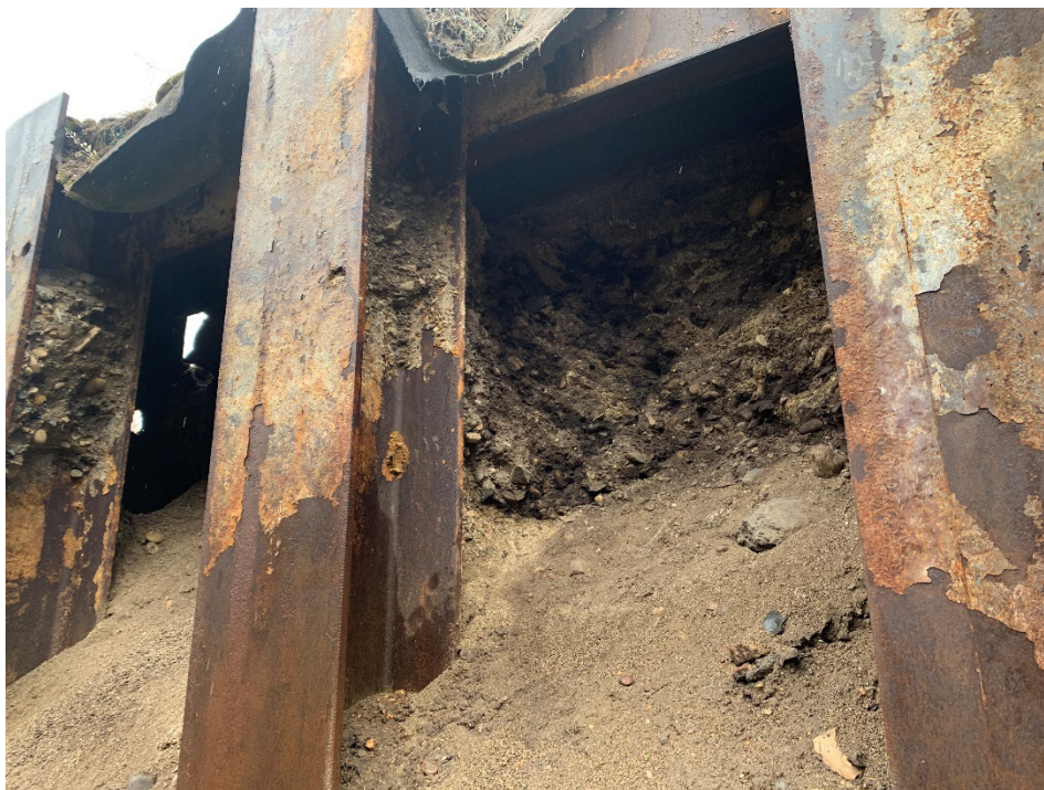
Photo 6 Site B: Erosion of material between piles has contributed to voids up to 0.5 m behind the wall. Photo taken facing northeast on May 11, 2023.
