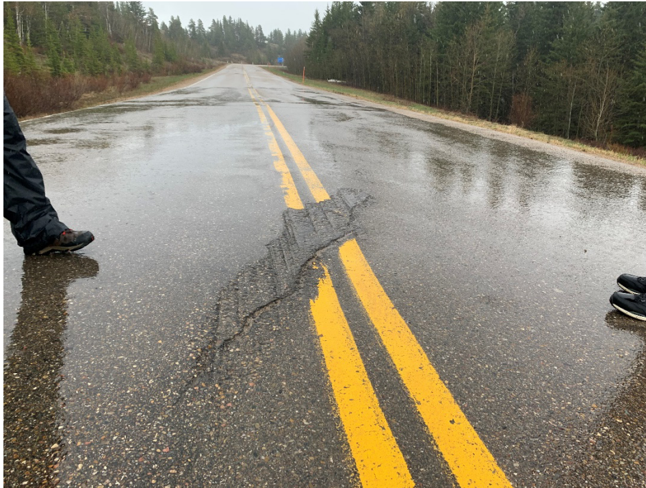
Photo 2 Site A: Pavement cracking and settlement. Photo was taken facing north on May 11, 2023.
