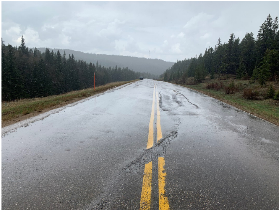
Photo 2 Site A: Pavement cracking and settlement. Photo was taken facing north on May 11, 2023.
