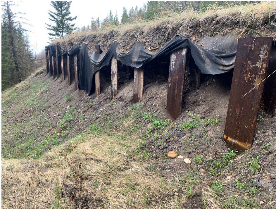
Photo 6 Site B: Erosion of material between piles has contributed to voids up to 0.5 m behind the wall. Photo taken facing northeast on May 11, 2023.
