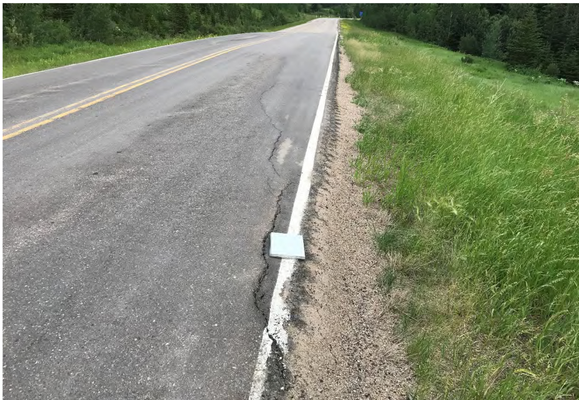
Photo 2 Site A: Pavement cracking. Photo was taken facing southeast on July 7, 2021.
