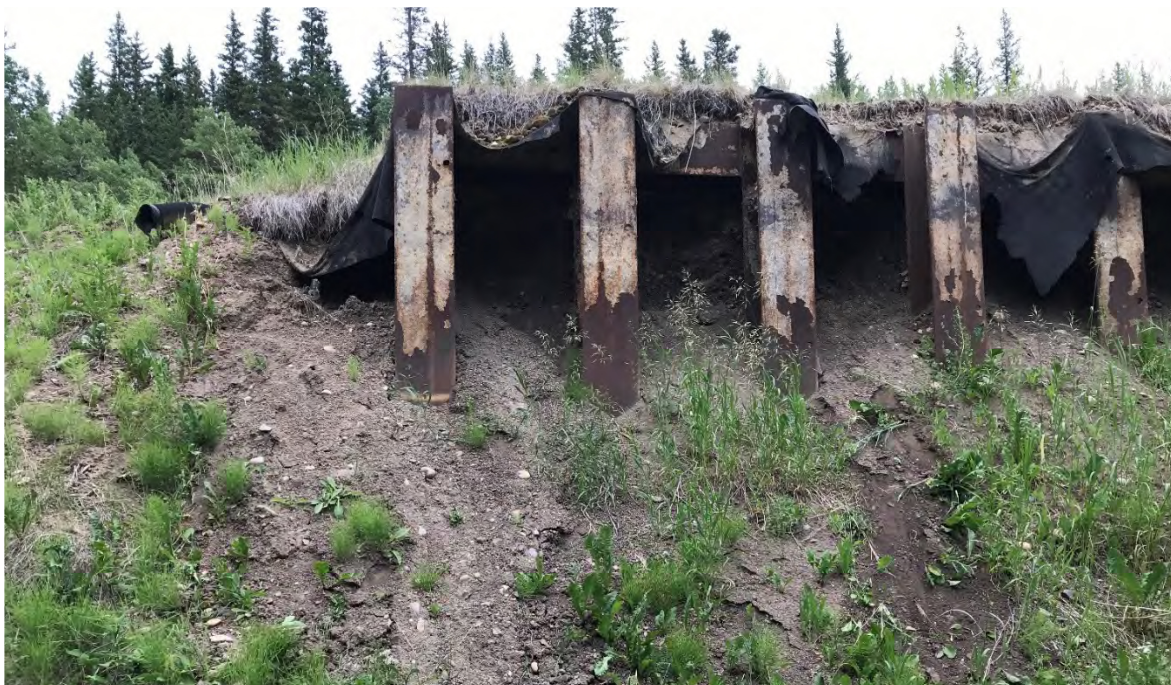
Photo 6 Site B: Erosion of material between piles has contributed to voids up to 0.5 m behind the wall. Photo taken facing north on July 7, 2021.
