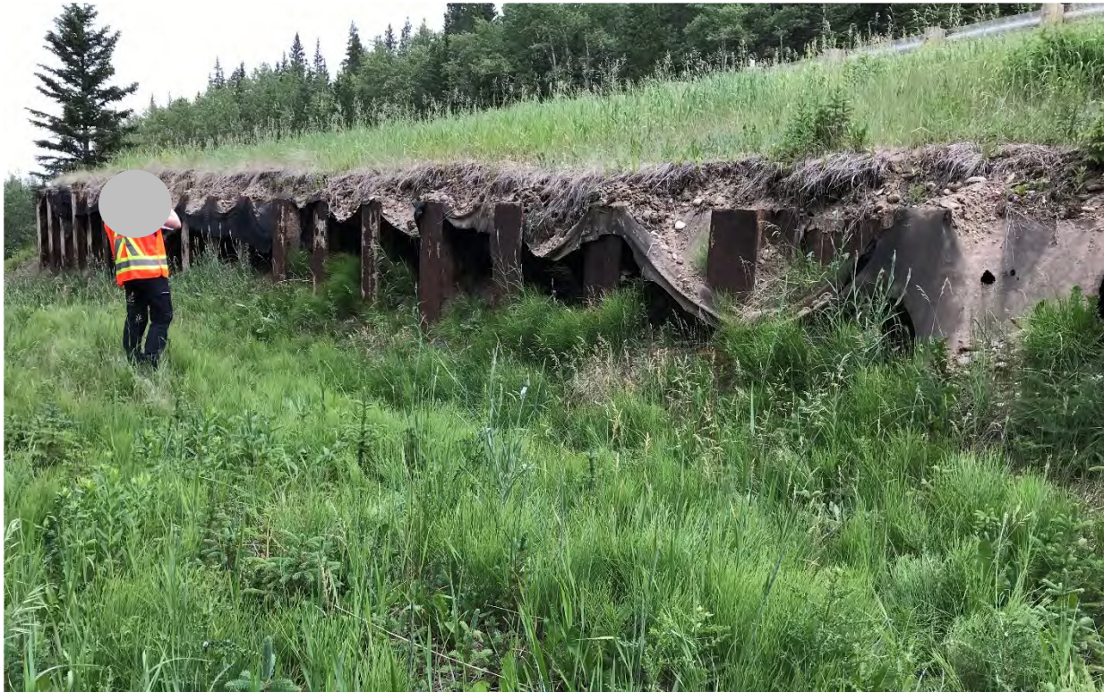
Photo 6 Site B: Erosion of material between piles has contributed to voids up to 0.5 m behind the wall. Photo taken facing north on July 7, 2021.
