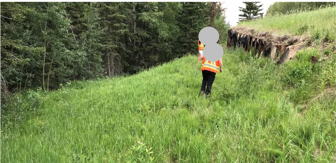
Photo 4 Site B: Pile wall is located downslope to the west of the highway. Soil sliding downslope of the wall has exposed 2 to 3 m of steel pile over a length of approximately 30 m. Photo was taken facing northwest on July 7, 2021.
