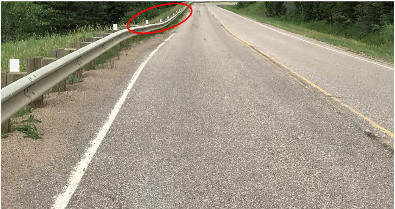
Photo 8 Site B: Dip in guard rail north of the pile wall. Photo taken facing north on July 7, 2021.
