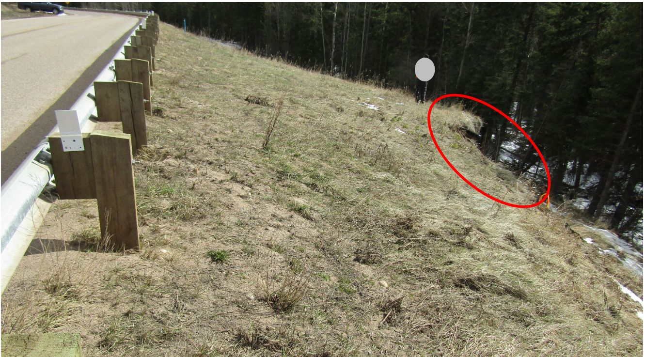
Photo 6 Back slope failure has blocked ditch, leading to standing water in ditch. Photo taken facing northeast on May 8, 2019.
