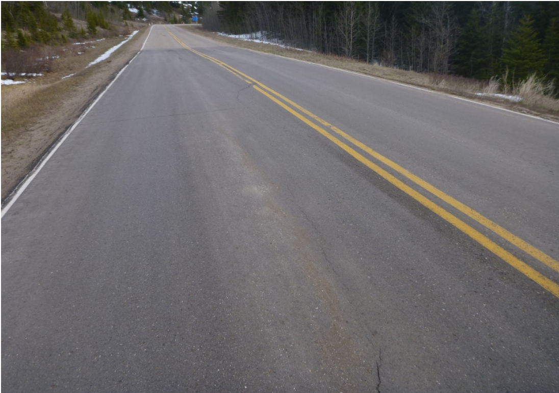
Photo 8 Pavement cracking and settlement at Site A. Photo taken on May 8, 2019.
