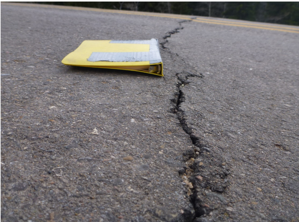
Photo 8 Pavement cracking and settlement at Site A. Photo taken on May 8, 2019.
