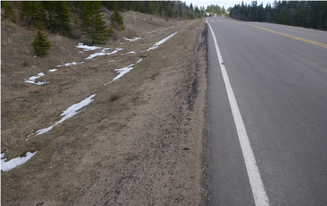
Photo 10 Back scarp of an embankment slide area, on the west slope at Area A site. Photo taken facing west on May 8, 2019.
