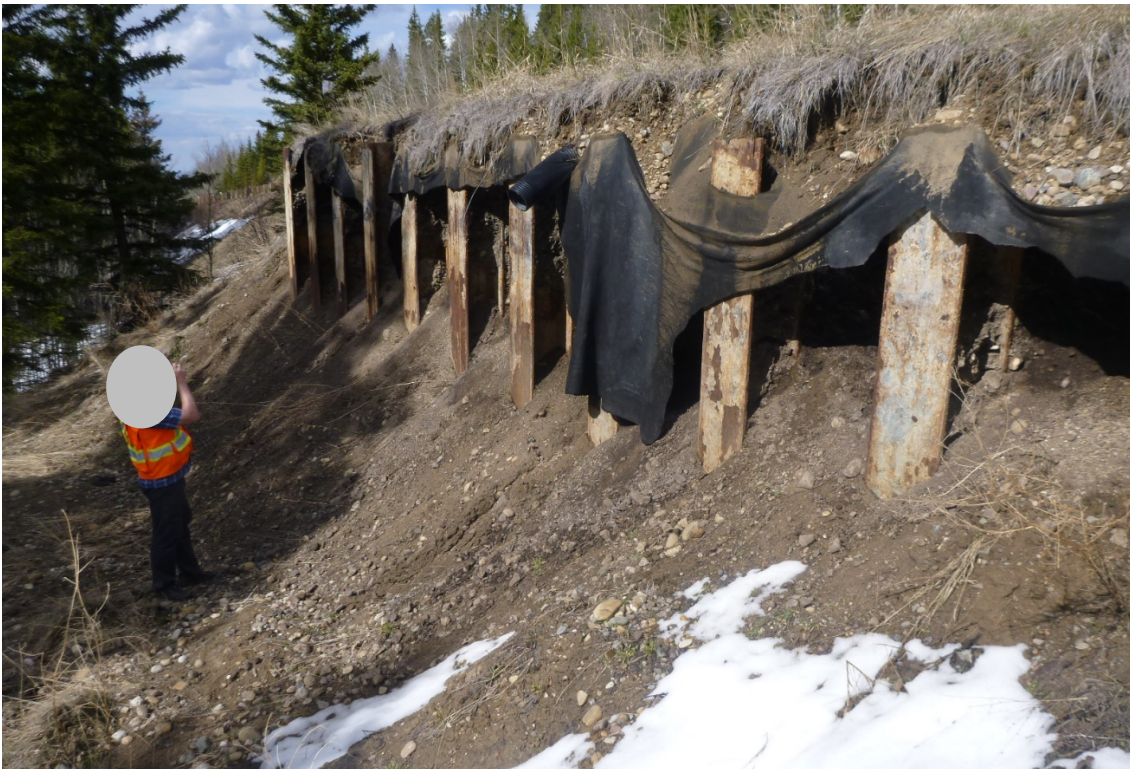
Photo 4 Exposed pile wall with 2 to 3 m of exposed H-pile and voids up to 0.5 m due to washout of material between piles. Photo taken facing north on May 8, 2019.
