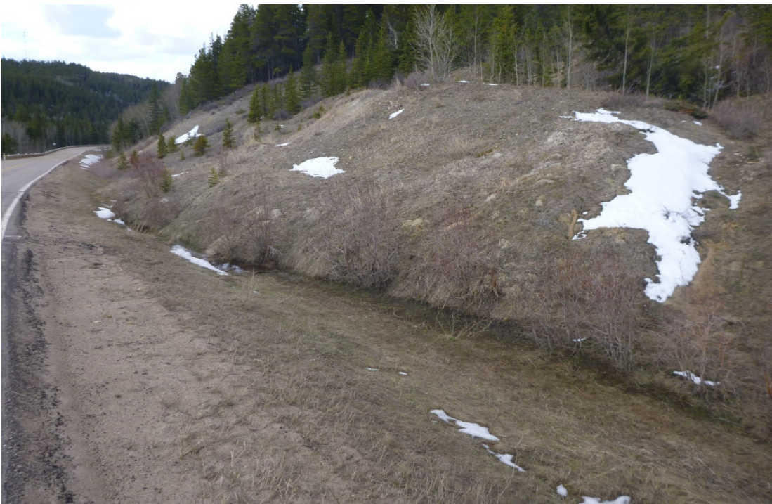
Photo 6 Back slope failure has blocked ditch, leading to standing water in ditch. Photo taken facing northeast on May 8, 2019.
