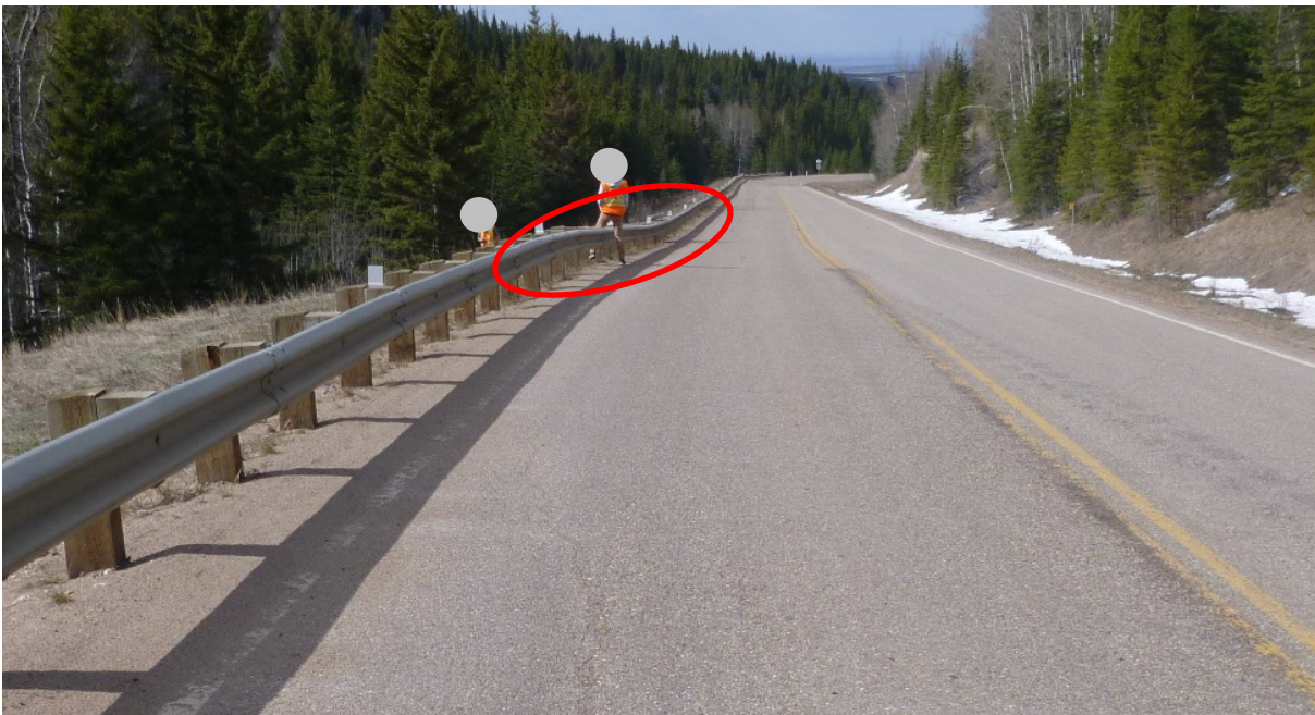
Photo 2 Dip in guard rail at Site B. Photo taken facing north on May 8, 2019.
