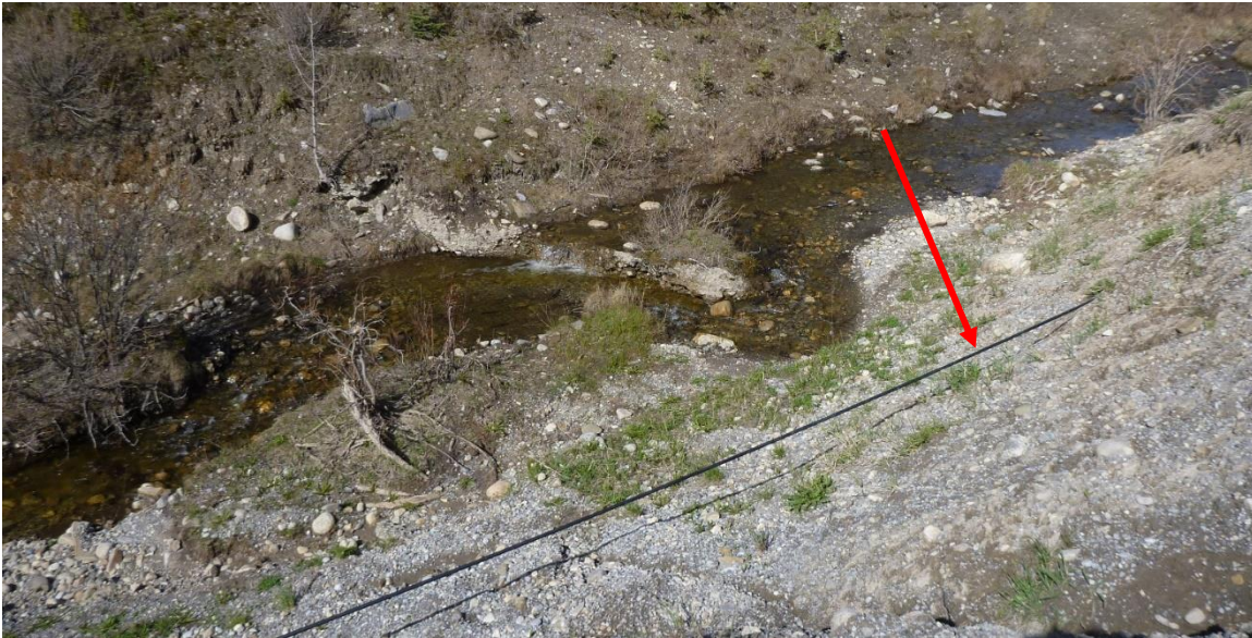
Photo 2 The erosion has retrogressed into the edge of the west (southbound) lane of highway. Photo taken May 27, 2024, facing south.
