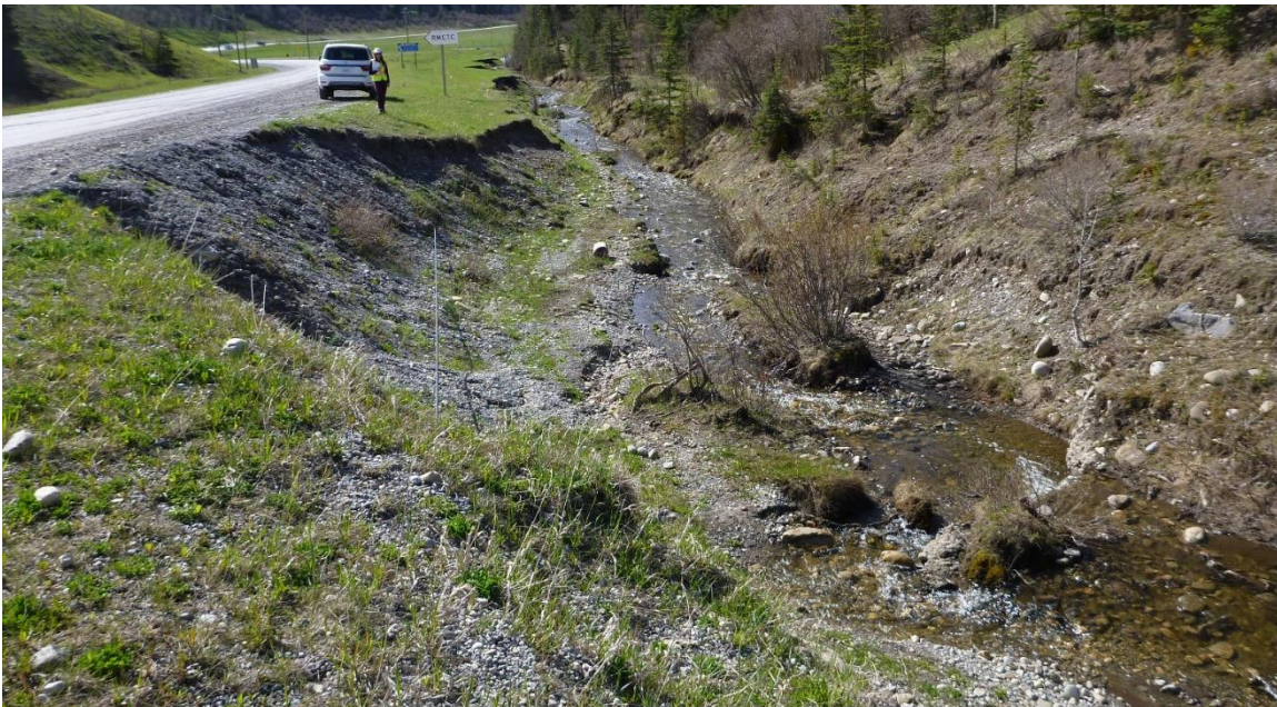
Photo 2 The erosion has retrogressed into the edge of the west (southbound) lane of highway. Photo taken May 27, 2024, facing south.
