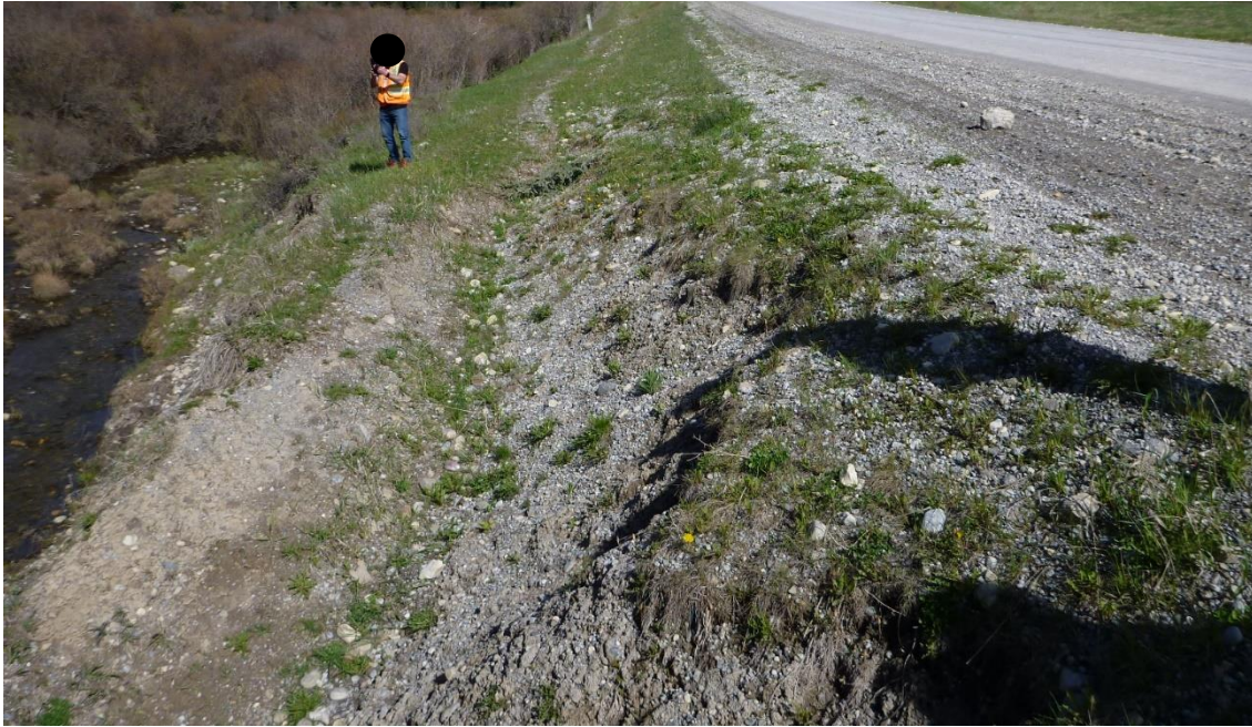
Photo 4 Erosion has retrogressed into the west shoulder for approximately 13 m along its length (indicated by red circle). Photo taken May 27, 2024, facing north.
