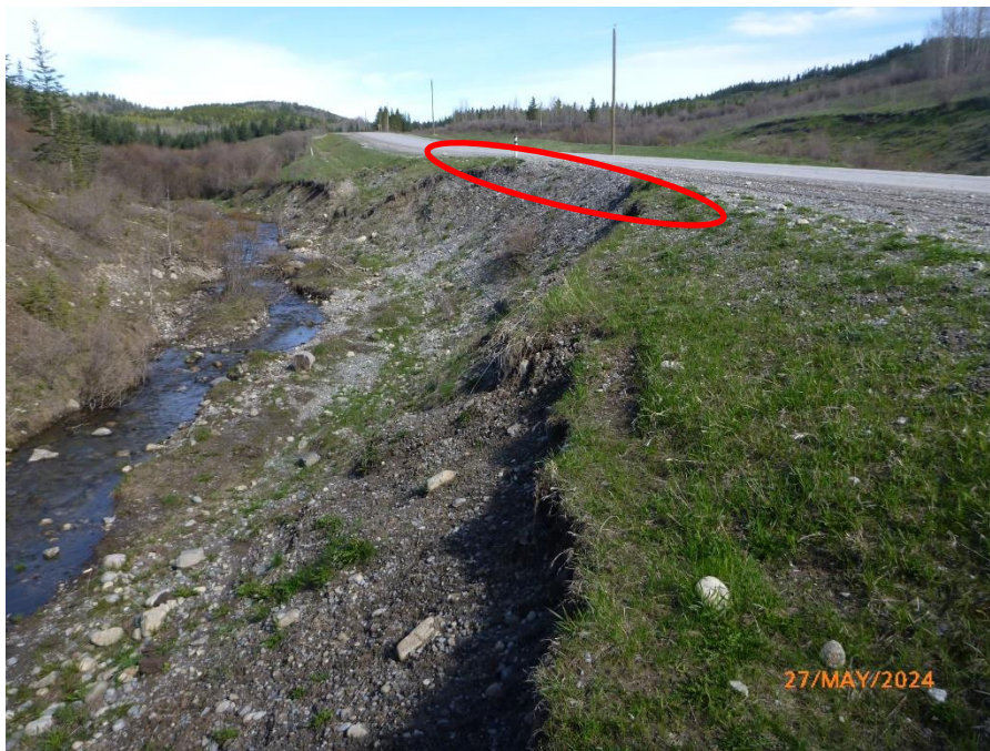
Photo 4 Erosion has retrogressed into the west shoulder for approximately 13 m along its length (indicated by red circle). Photo taken May 27, 2024, facing north.
