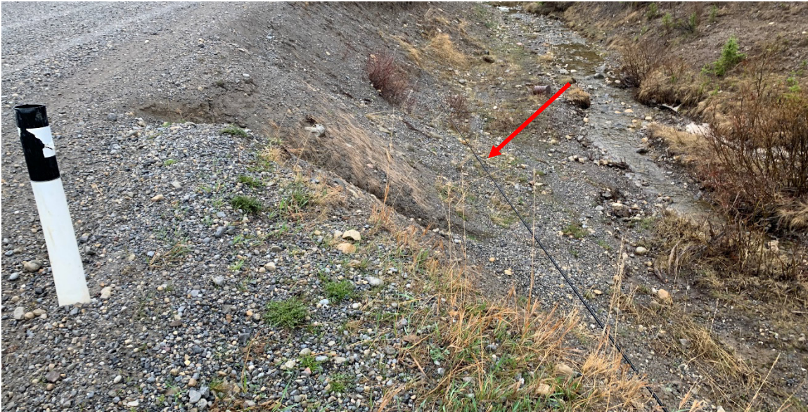
Photo 2 The erosion has retrogressed into the edge of the south (eastbound) lane of highway. Photo taken May 8, 2023, facing southeast.
