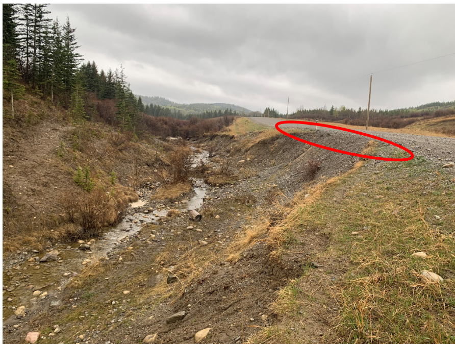
Photo 4 The erosion of the south highway embankment has exposed a black utility cable and has over-steepened the highway embankment (approximately 1H:1V). Erosion has retrogressed into the south shoulder for approximately 13 m along its length (Where indicated by red circle). Photo taken May 8, 2023, facing northwest.
