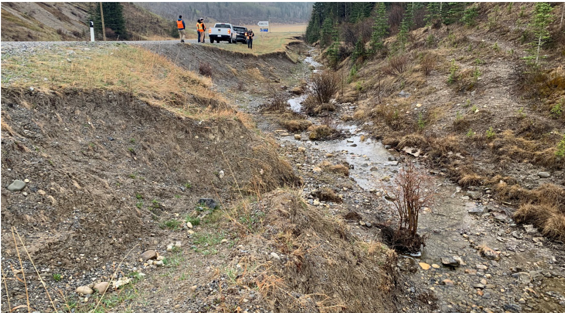
Photo 2 The erosion has retrogressed into the edge of the south (eastbound) lane of highway. Photo taken May 8, 2023, facing southeast.
