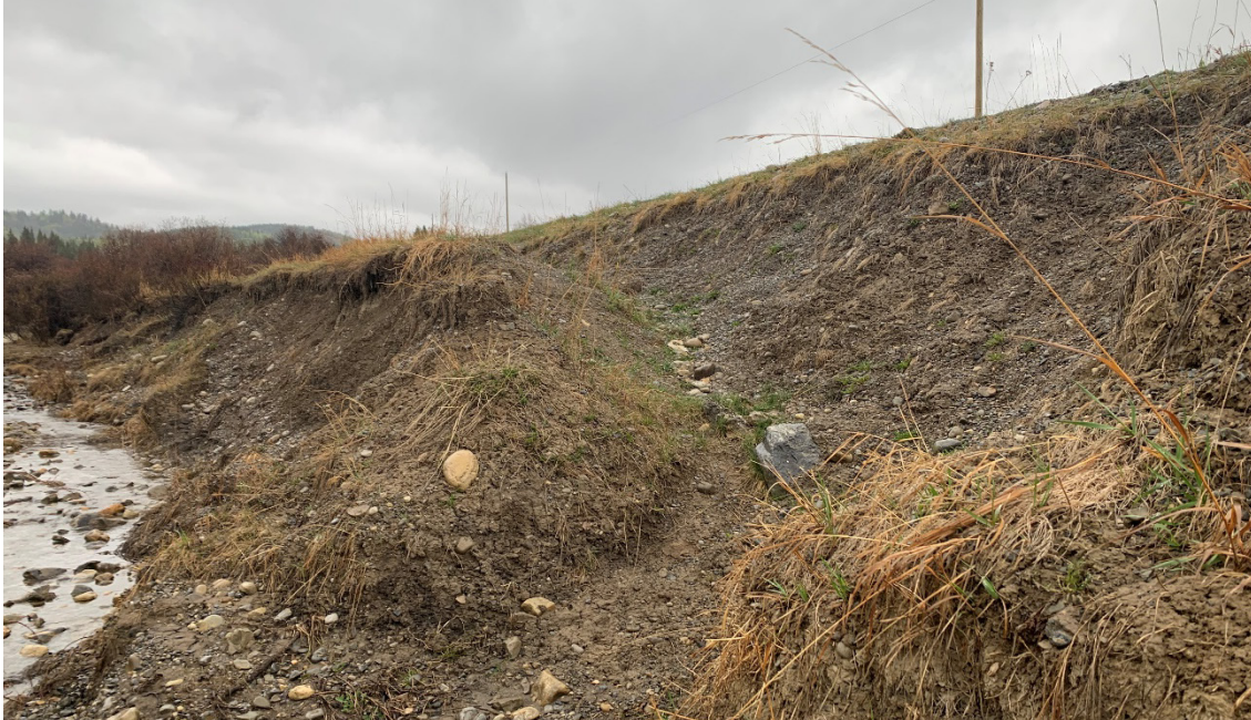
Photo 4 The erosion of the south highway embankment has exposed a black utility cable and has over-steepened the highway embankment (approximately 1H:1V). Erosion has retrogressed into the south shoulder for approximately 13 m along its length (Where indicated by red circle). Photo taken May 8, 2023, facing northwest.
