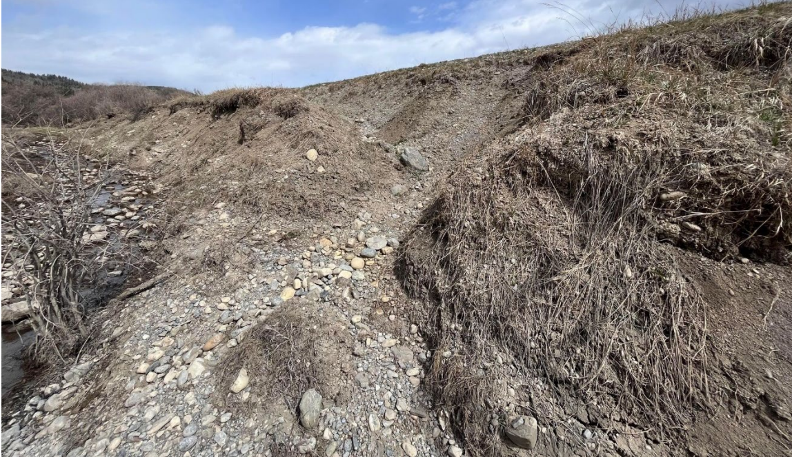
Photo 4 The erosion of the south highway embankment has exposed a black utility cable (indicated by black arrow) and has over-steepened the highway embankment (approximately 1H:1V). Photo taken May 18, 2022, facing northwest.
