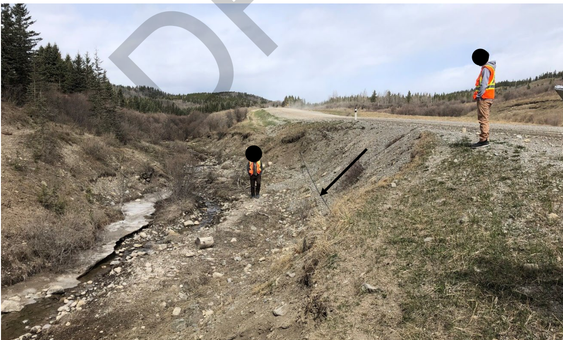
Photo 4 The erosion of the south highway embankment has exposed a black utility cable (indicated by black arrow) and has over-steepened the highway embankment (approximately 1H:1V). Photo taken May 18, 2022, facing northwest.
