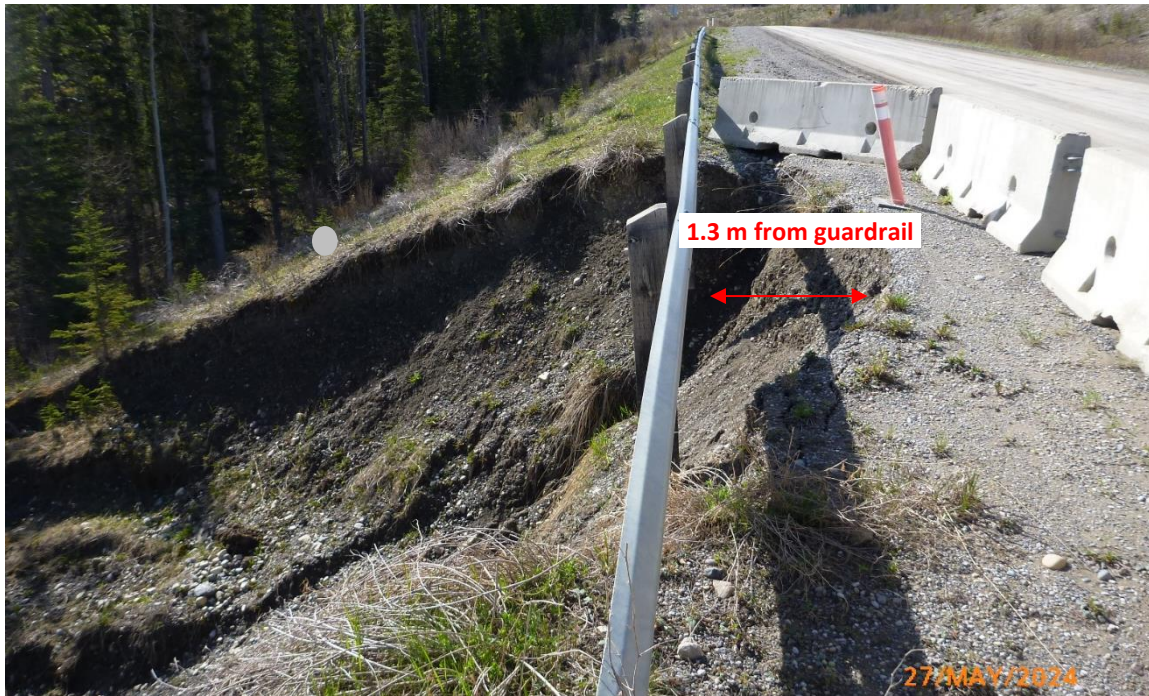
Photo 2 View from highway down the erosion gully and separated culvert. Photo taken facing east on May 27, 2024.
