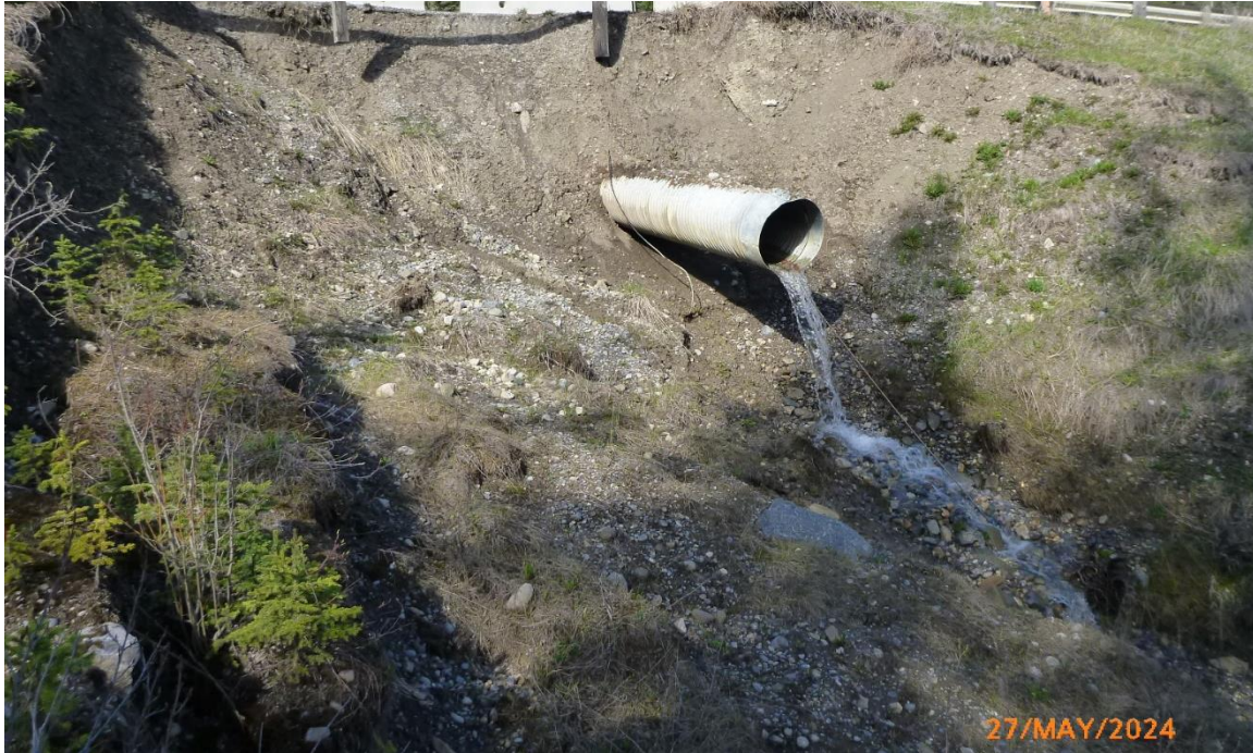
Photo 4 Separated culvert and trees felled in the erosion site. Photo taken facing northeast on May 27, 2024.
