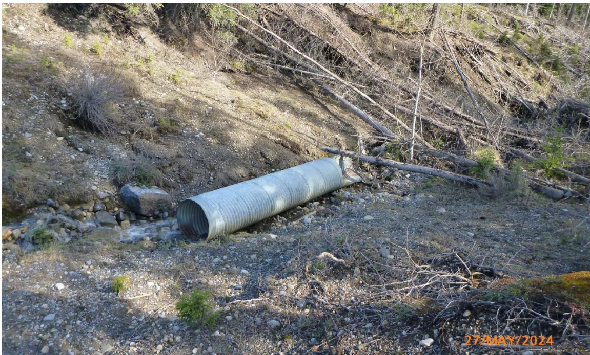
Photo 4 Separated culvert and trees felled in the erosion site. Photo taken facing northeast on May 27, 2024.
