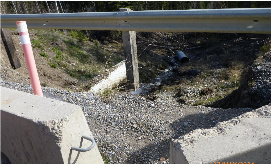
Photo 2 View from highway down the erosion gully and separated culvert. Photo taken facing east on May 27, 2024.
