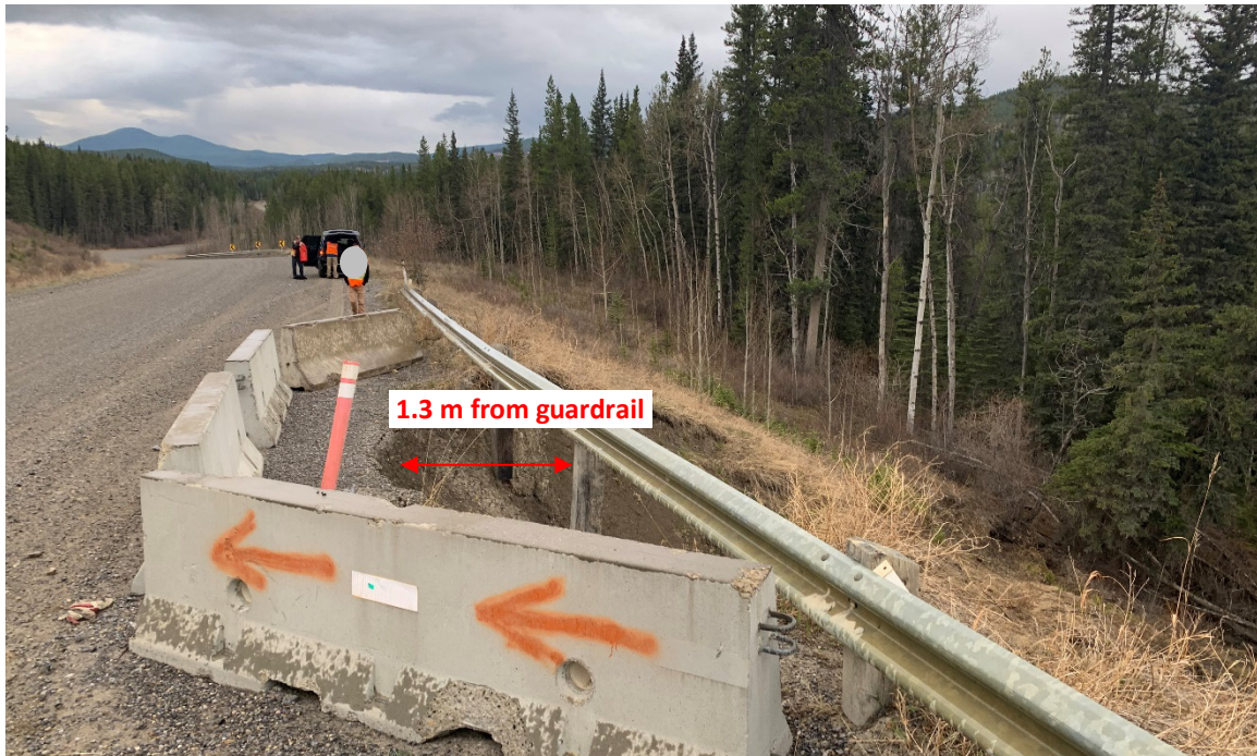
Photo 2 View from highway down the erosion gully and separated culvert. Photo taken facing east on May 8, 2023.
