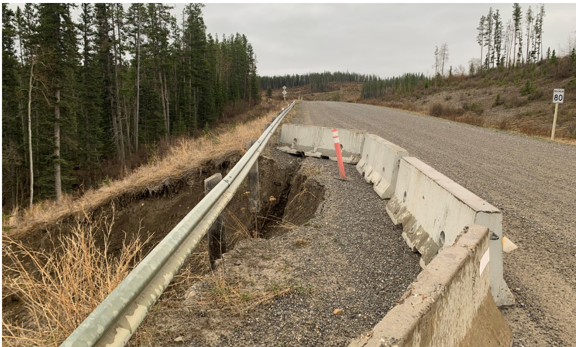
Photo 4 Barriers placed around the erosion into the road. Photo taken facing south on May 8, 2023.
