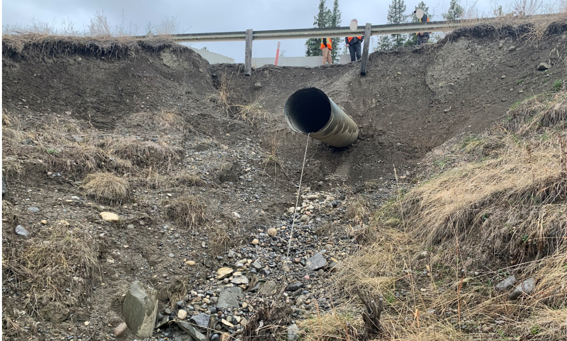
Photo 4 Barriers placed around the erosion into the road. Photo taken facing south on May 8, 2023.
