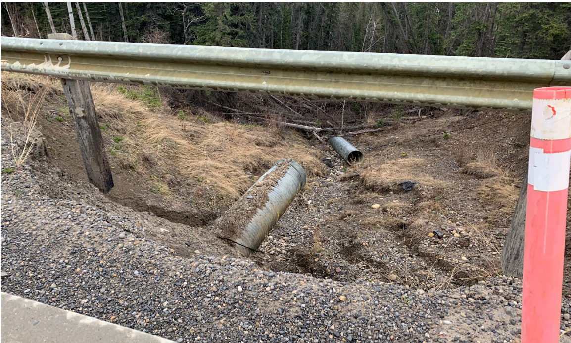
Photo 2 View from highway down the erosion gully and separated culvert. Photo taken facing east on May 8, 2023.
