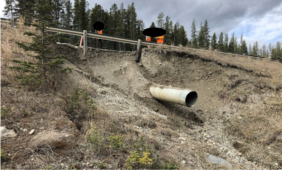
Photo 4 Delineator used to mark the location of where the erosion is retrogressing into the gravel road surface. Photo taken May 18, 2022 facing northwest.
