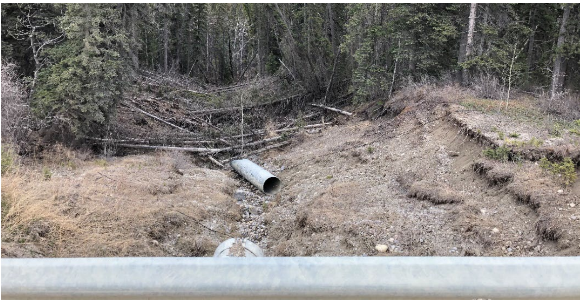
Photo 2 View from highway down the erosion gully and toward the separated culvert. Photo taken May 18, 2022, facing northeast.
