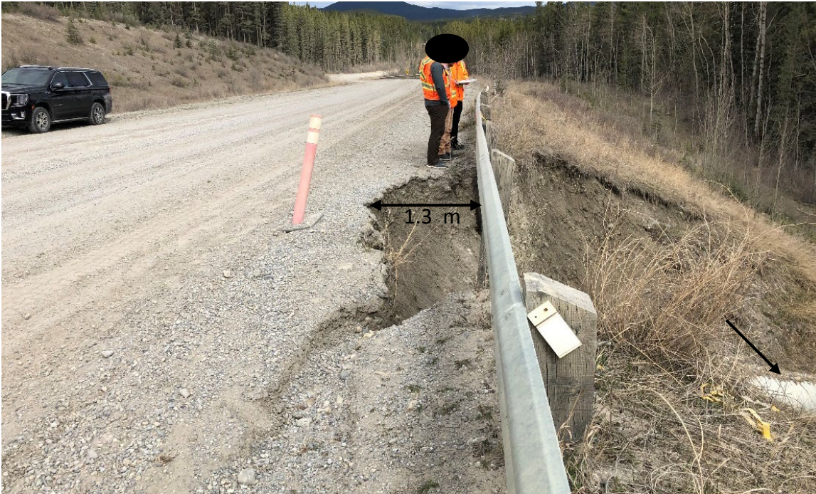
Photo 2 View from highway down the erosion gully and toward the separated culvert. Photo taken May 18, 2022, facing northeast.
