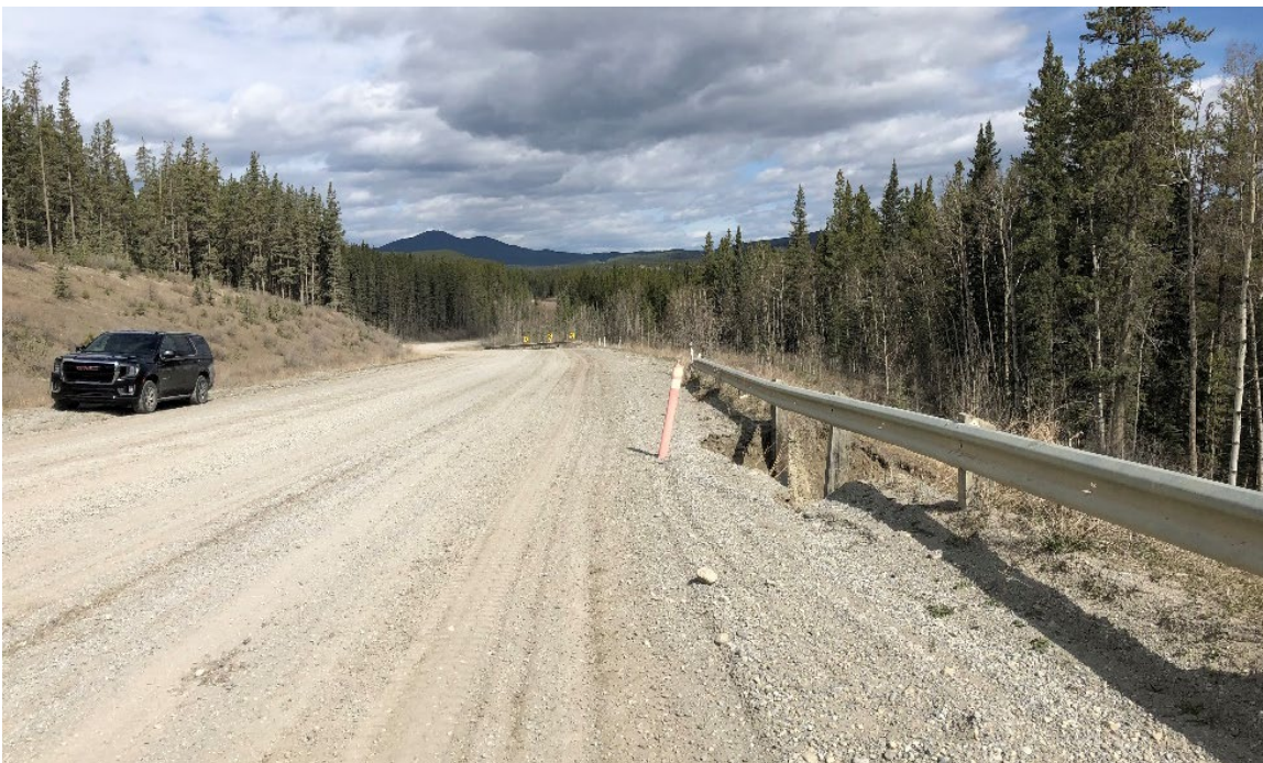
Photo 4 Delineator used to mark the location of where the erosion is retrogressing into the gravel road surface. Photo taken May 18, 2022 facing northwest.
