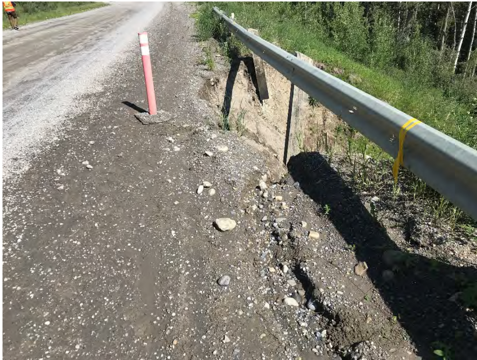
Photo 2 View from highway down the erosion gully and separated culvert. Photo taken facing northeast on July 6, 2021.
