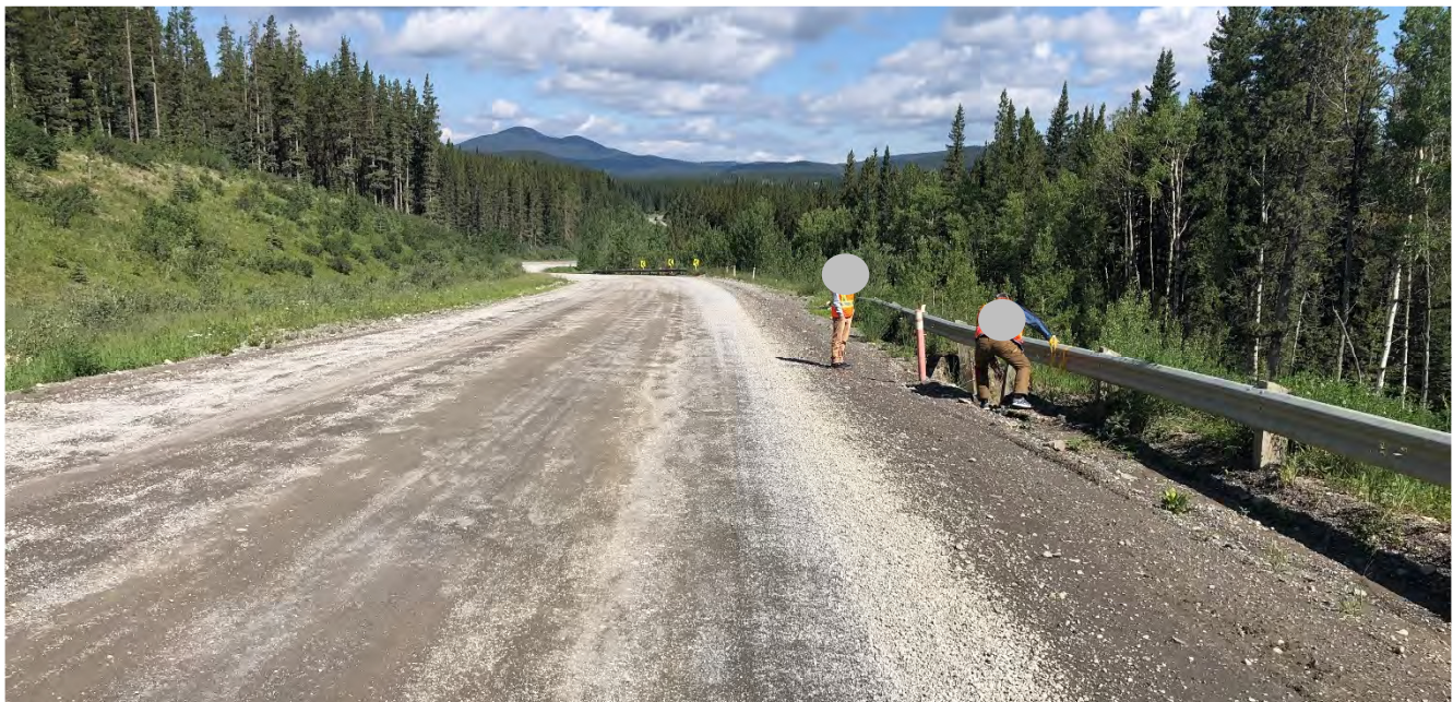
Photo 4 Delineator used to mark erosion retrogressing into the gravel road surface. Photo taken facing northwest on July 6, 2021.
