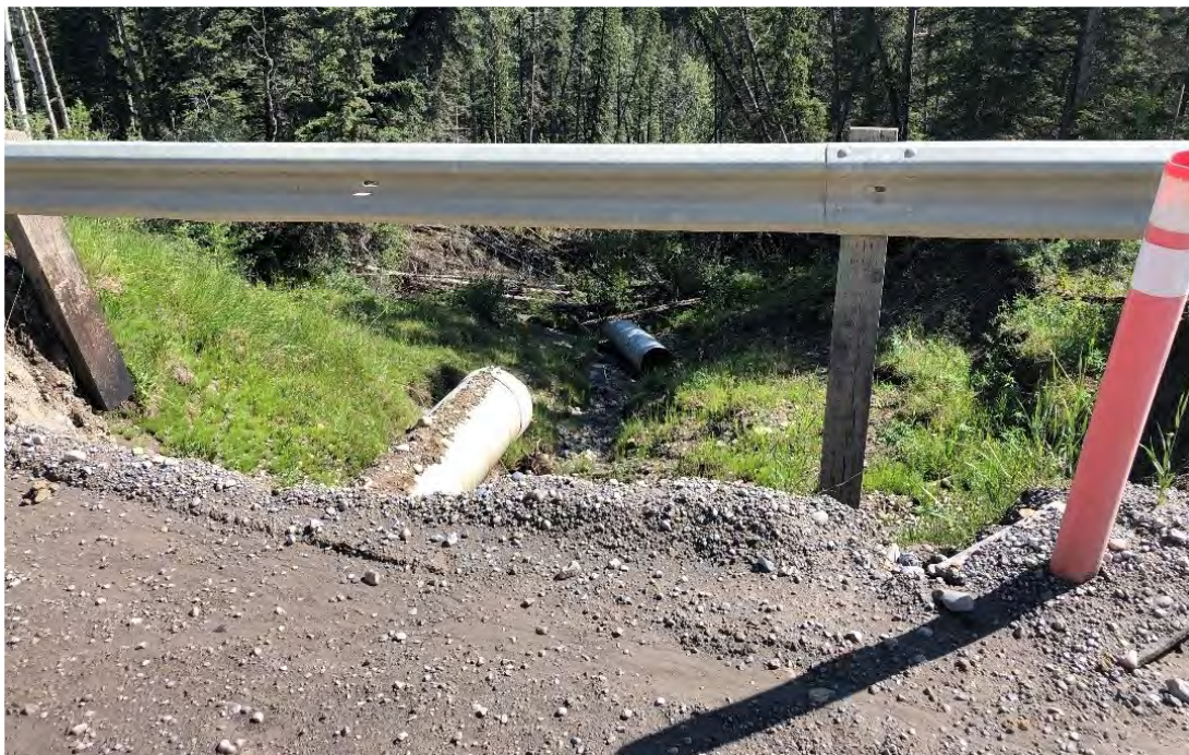
Photo 2 View from highway down the erosion gully and separated culvert. Photo taken facing northeast on July 6, 2021.
