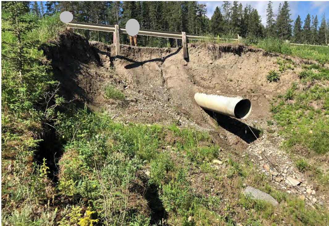
Photo 4 Delineator used to mark erosion retrogressing into the gravel road surface. Photo taken facing northwest on July 6, 2021.
