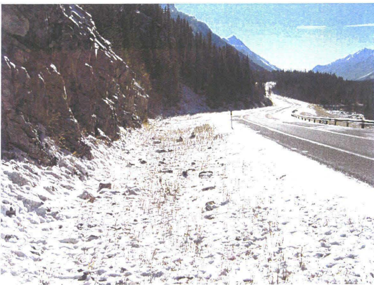
Photo 2 (bottom) – Facing south along Highway 40 at the Limestone Mountain Cut Slope site. Some segments of the cut slope at this site experience rockfall originating from the steep soil/rock slope above the crest of the near-vertical, lower cut slope. As shown in this photo, the rockfall debris is contained within the existing ditch.
