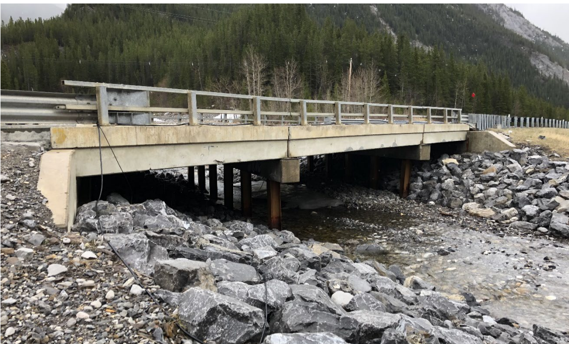
Photo 2 Upstream side of Rocky Creek Bridge. The upstream H-piles appear partially displaced from a suspected high-water event. Photo taken May 17, 2022, facing east.
