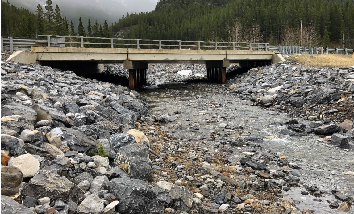
Photo 2 Upstream side of Rocky Creek Bridge. The upstream H-piles appear partially displaced from a suspected high-water event. Photo taken May 17, 2022, facing east.
