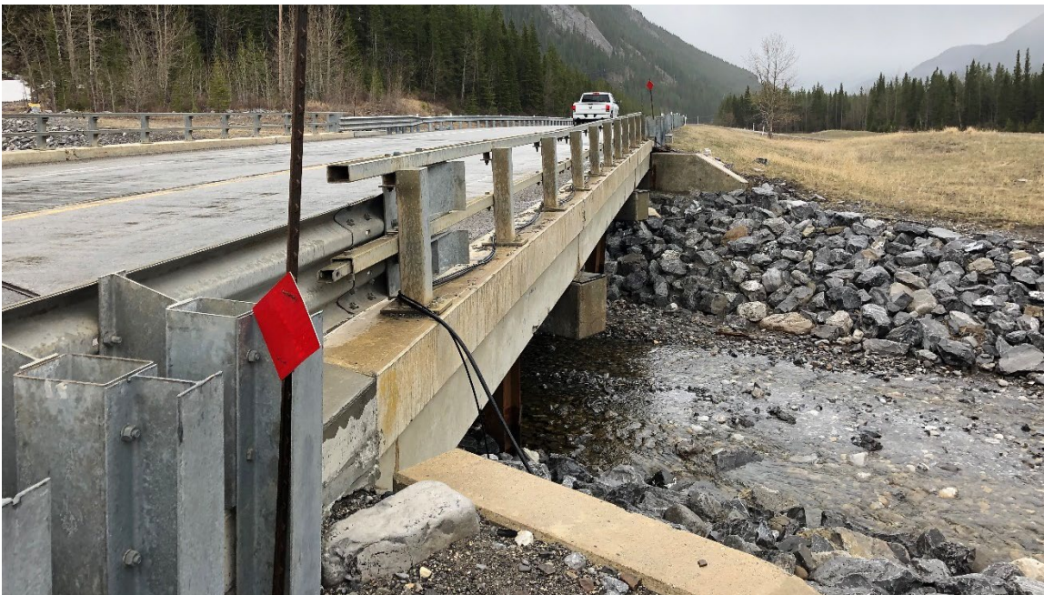
Photo 4 The pavement north/south and above the Rocky Creek Bridge appears to be in good condition. Guardrails have been installed along the east and west sides of the highway leading up to and along the bridge. Photo taken May 17, 2022, facing south.
