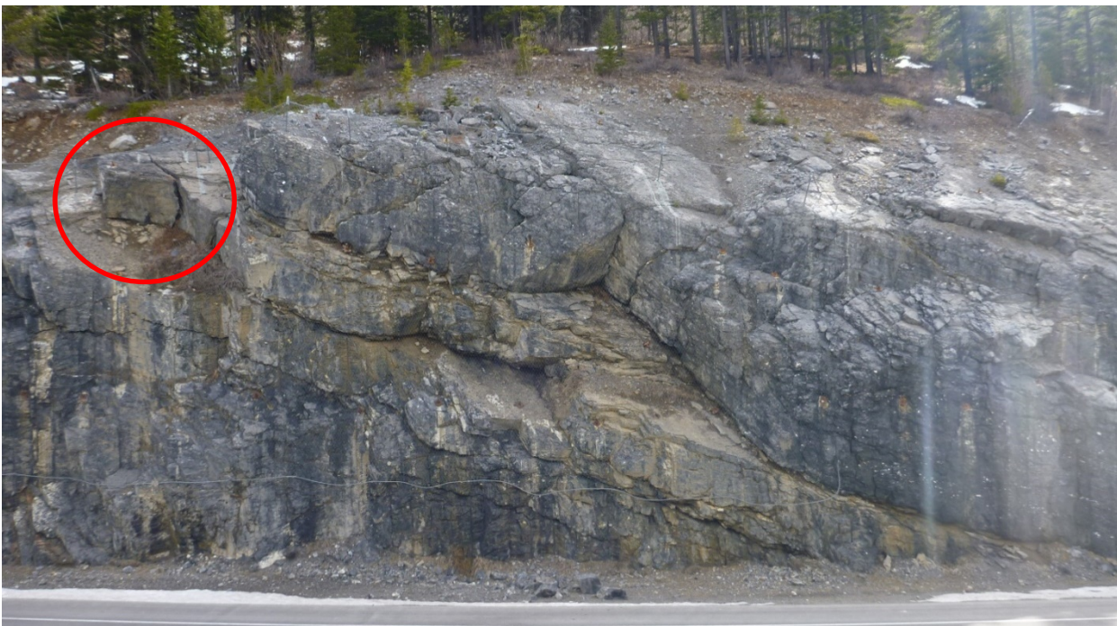
Photo 4 Central portion of east rock slope, including large block held by an off-centre rock bolt. Photo taken facing southeast on May 7, 2019.
