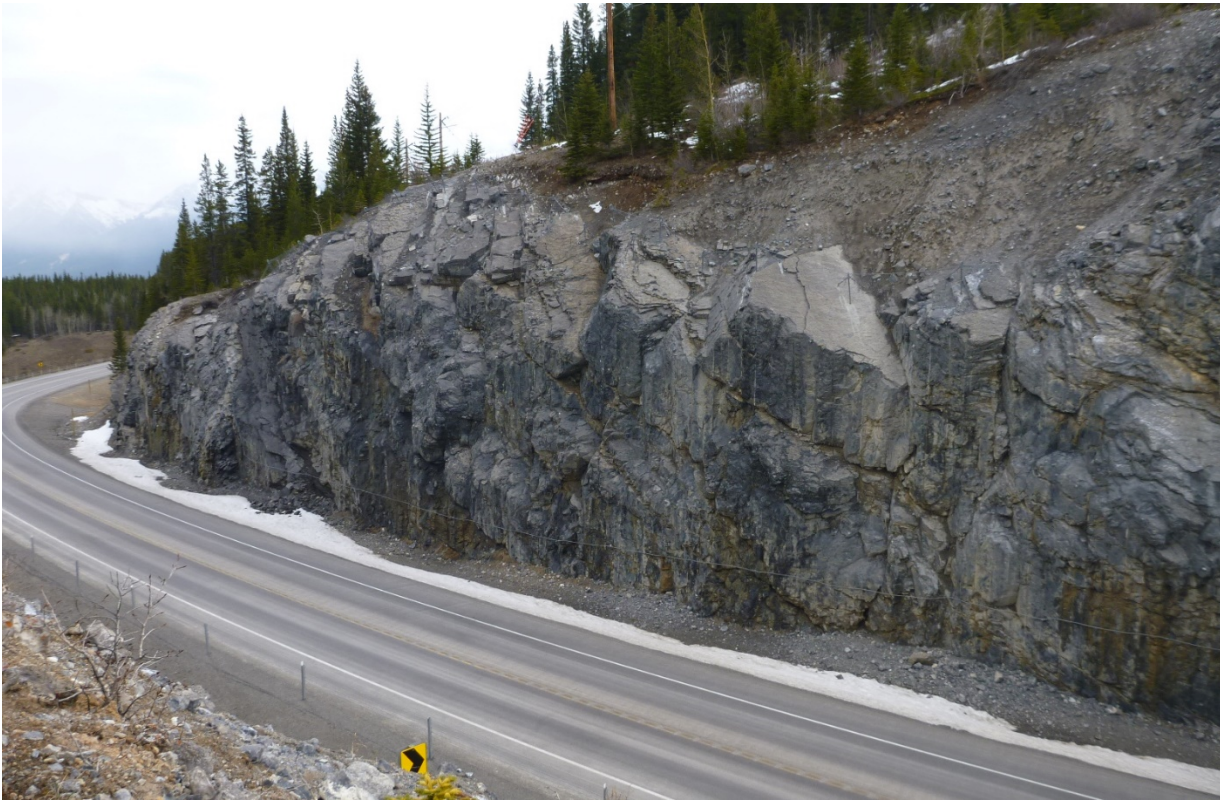
Photo 4 Central portion of east rock slope, including large block held by an off-centre rock bolt. Photo taken facing southeast on May 7, 2019.
