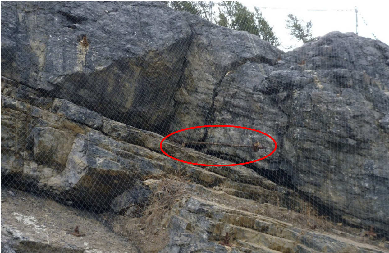
Photo 6 Damaged connections between the wire mesh and base cable due to rockfall impacts. Photo taken on May 7, 2019.
