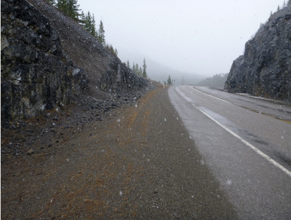
Photo 3 Rock debris in west ditch. Photo was taken facing northeast on May 1, 2018.
