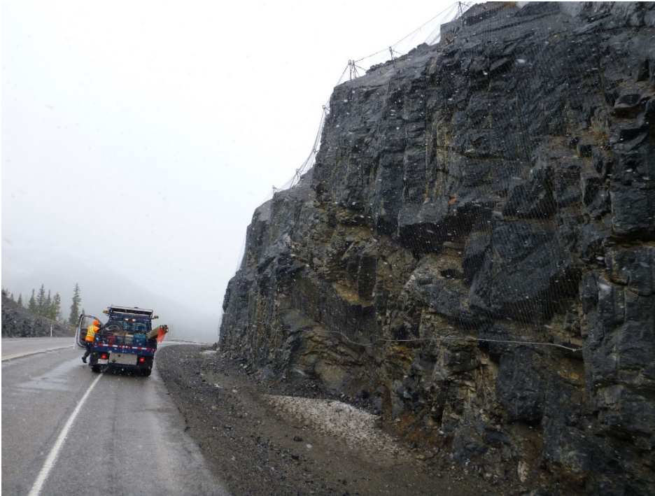
Photo 2 Recent rock fall of about 1 m 3 from approximately 2 m above ground, behind wire mesh. Photo was taken facing east on May 1, 2018.
