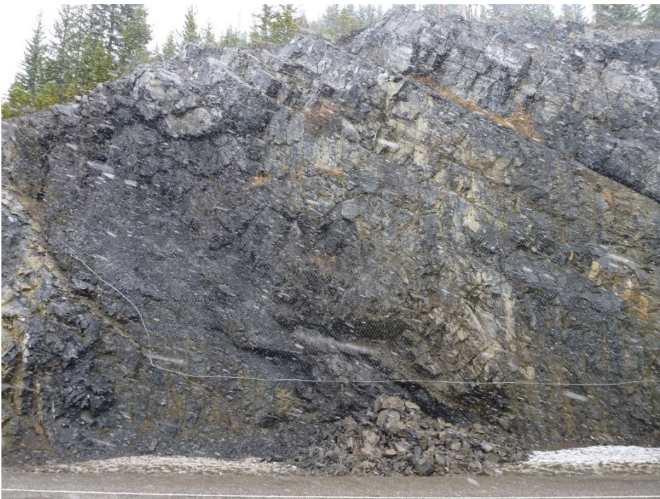
Photo 2 Recent rock fall of about 1 m 3 from approximately 2 m above ground, behind wire mesh. Photo was taken facing east on May 1, 2018.
