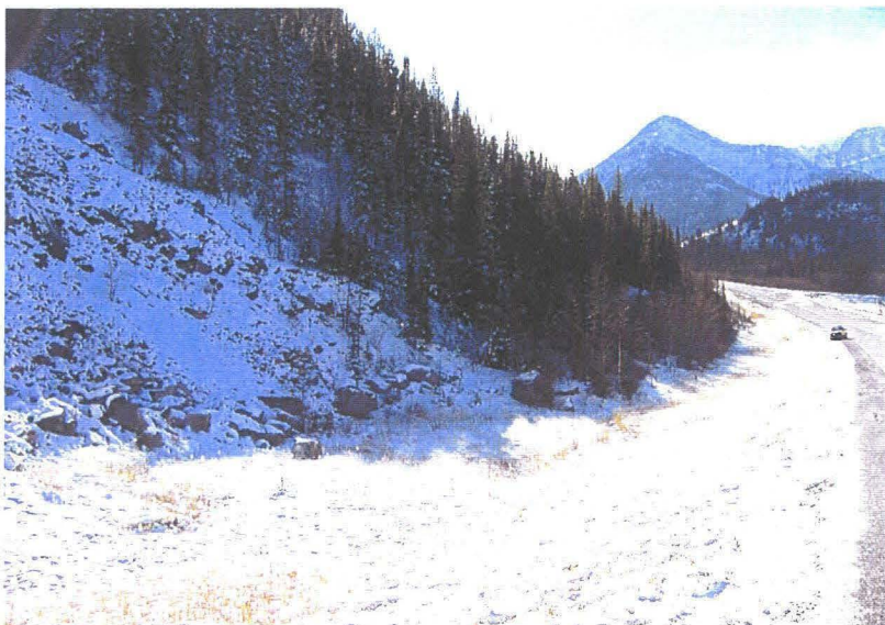
Photo 1 (top) – The Barrier Bluffs rock slope above Highway 40. The highway is located adjacent to the toe of a colluvium slope below a near-vertical rock slope. The colluvium slope is at an angle of around 35°. The ditch between the highway and the toe of the colluvium has a minimum width of approximately 10 m and a depth of approximately 3 to 4 m relative to the road surface.
