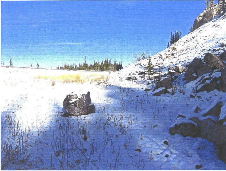
Photo 3 (top) – Large boulder that has rolled beyond the toe of the colluvium slope and come to rest in the central portion of the ditch along the highway.
