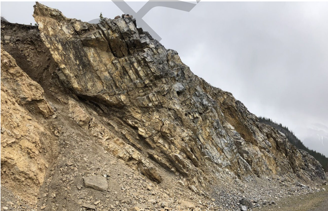
Photo 4 At the south end of the east rockfall site there is more severe weathering along the bedding planes leading to more overhangs that could lead to more rockfall debris. Photo taken May 17, 2022, facing southwest.
