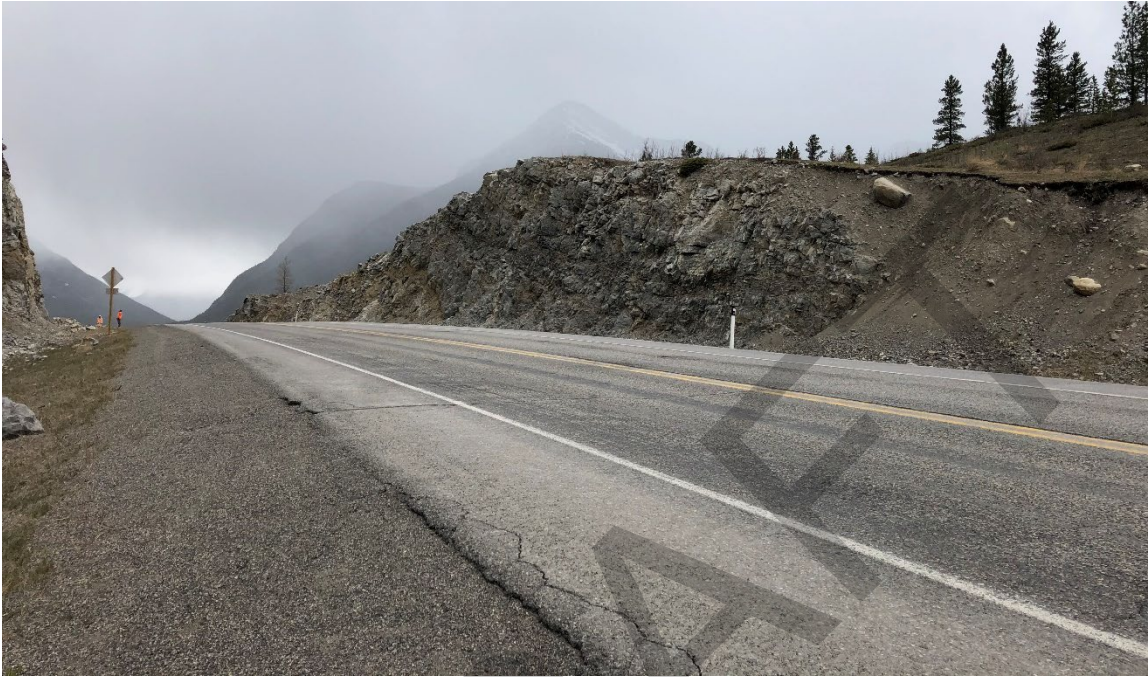
Photo 6 The west (southbound) ditch is approximately 0.8 m to 1.0 m deep and 3 m wide and has more rockfall capacity than the east (northbound) ditch. Photo taken May 17, 2022, facing southwest.
