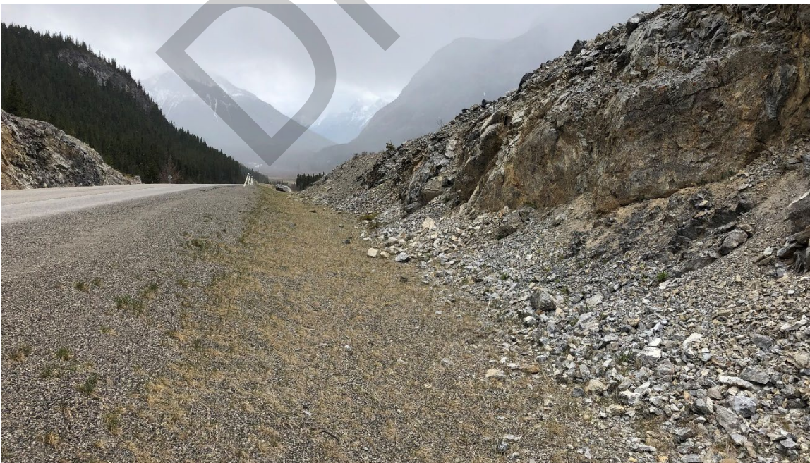
Photo 6 The west (southbound) ditch is approximately 0.8 m to 1.0 m deep and 3 m wide and has more rockfall capacity than the east (northbound) ditch. Photo taken May 17, 2022, facing southwest.
