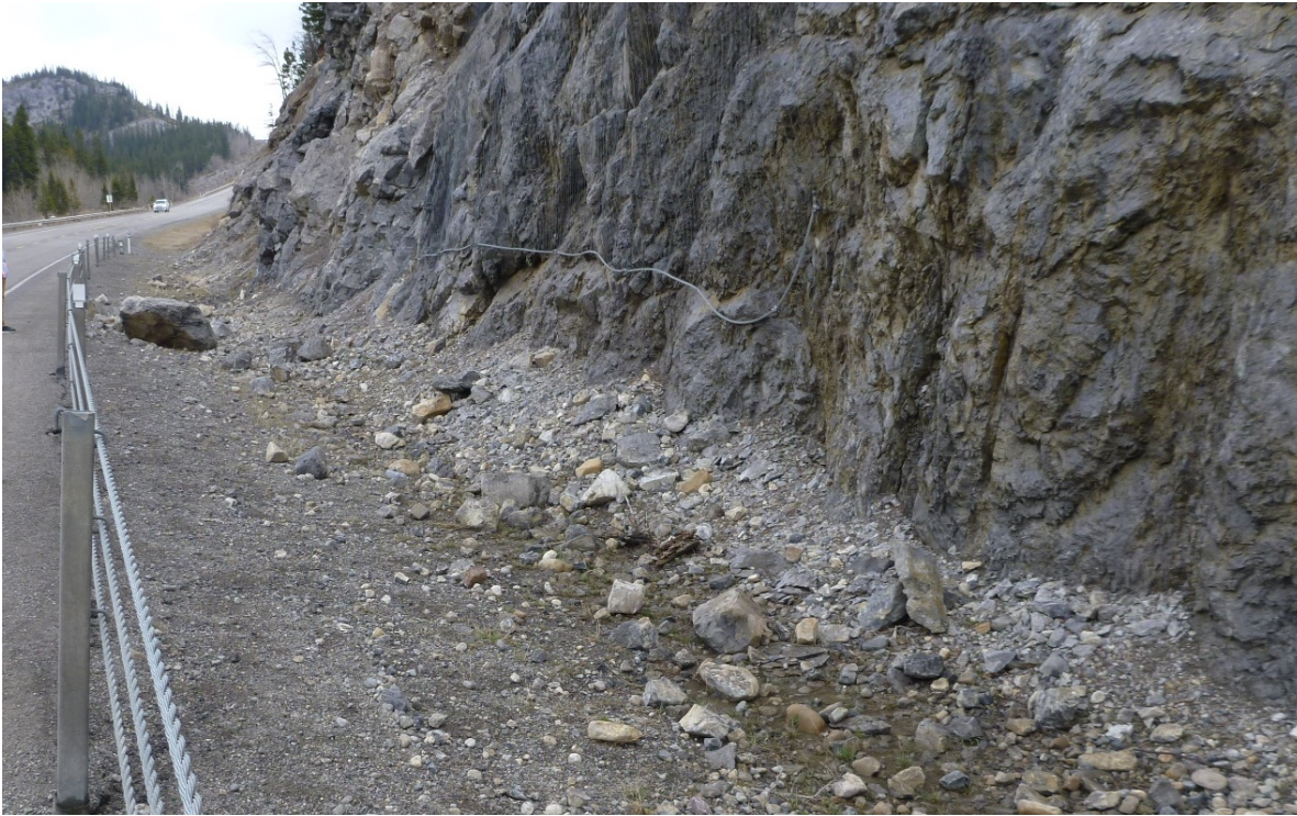
Photo 4 Some tears noted in the wire mesh where attached to the cable at the base. Photo was taken on May 7, 2019.
