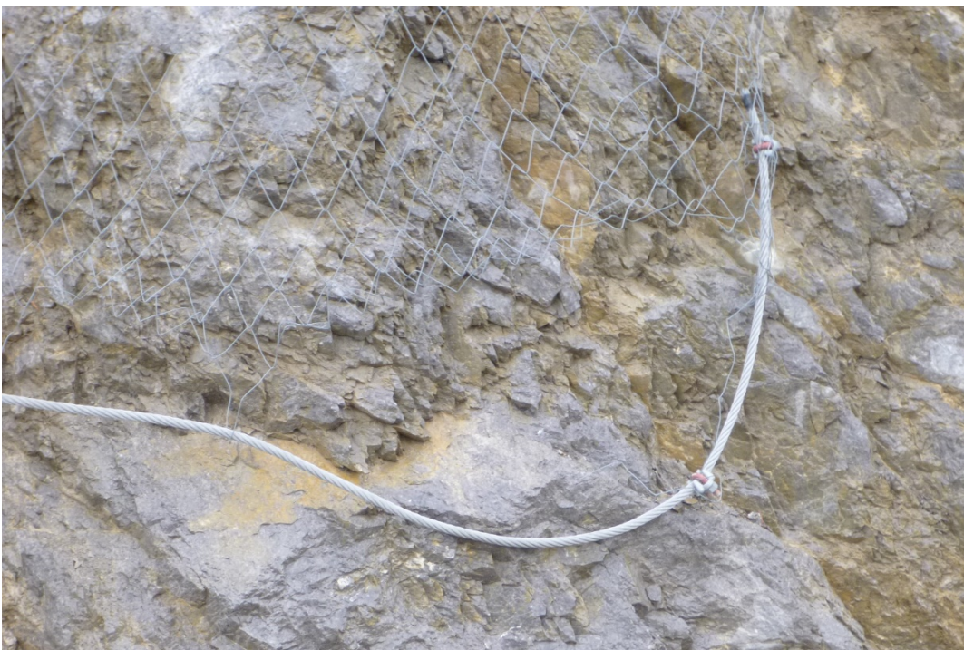
Photo 4 Some tears noted in the wire mesh where attached to the cable at the base. Photo was taken on May 7, 2019.
