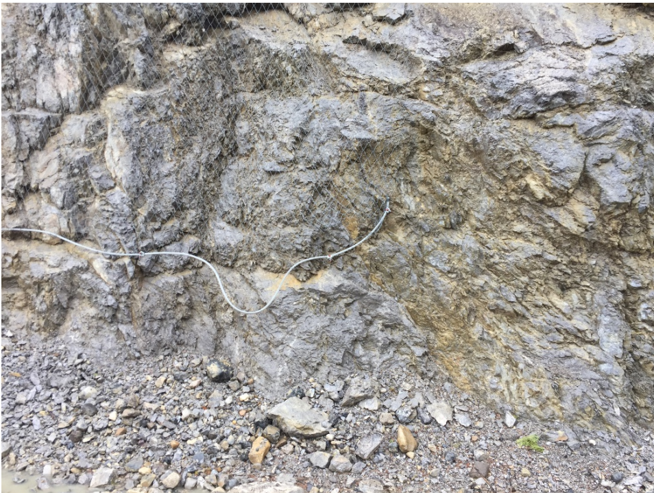
Photo 4 Some tears noted in the wire mesh where attached to the cable at the base. Photo was taken facing east on May 1, 2018.
