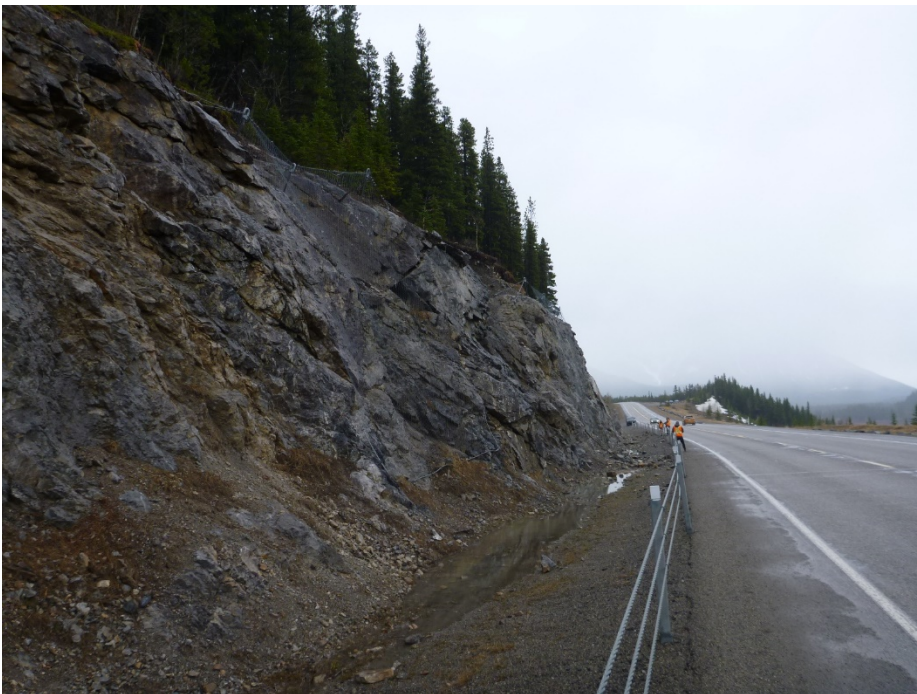
Photo 2 Wire mesh and HTC B installed on slope in 2016. Photo was taken facing south on May 1, 2018.
