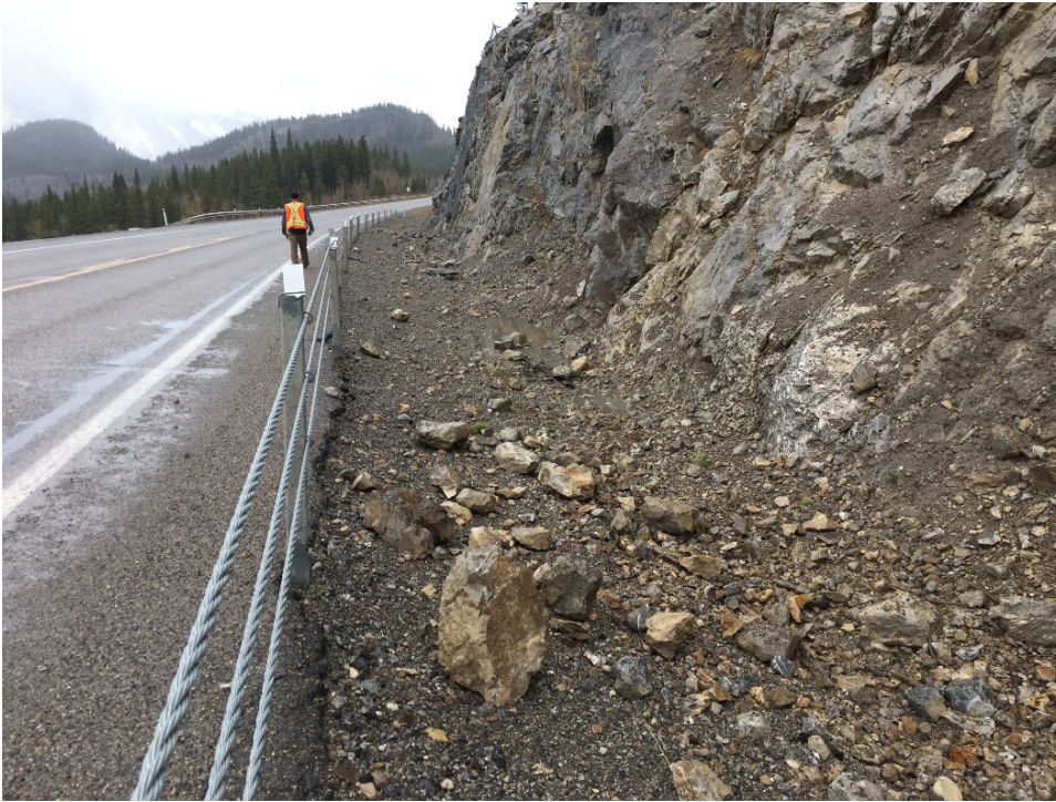
Photo 4 Some tears noted in the wire mesh where attached to the cable at the base. Photo was taken facing east on May 1, 2018.
