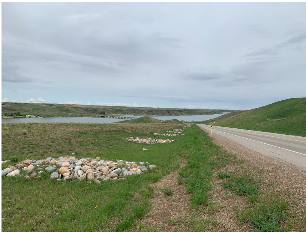
Photo 4 Ditch check dams. Photo taken facing west on May 11, 2023.
