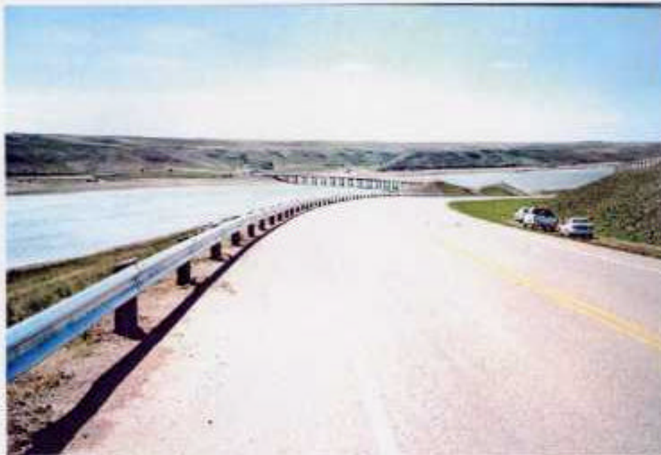
Photo 4 – Facing southwest along road through slide area. Note newly-installed guardrail.
