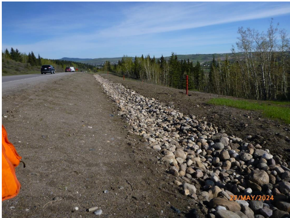
Photo 2 North end of the project area with the ditch reinstated with riprap. Pile wall installed downslope of ditch. Photo was taken facing northwest on May 27, 2024.
