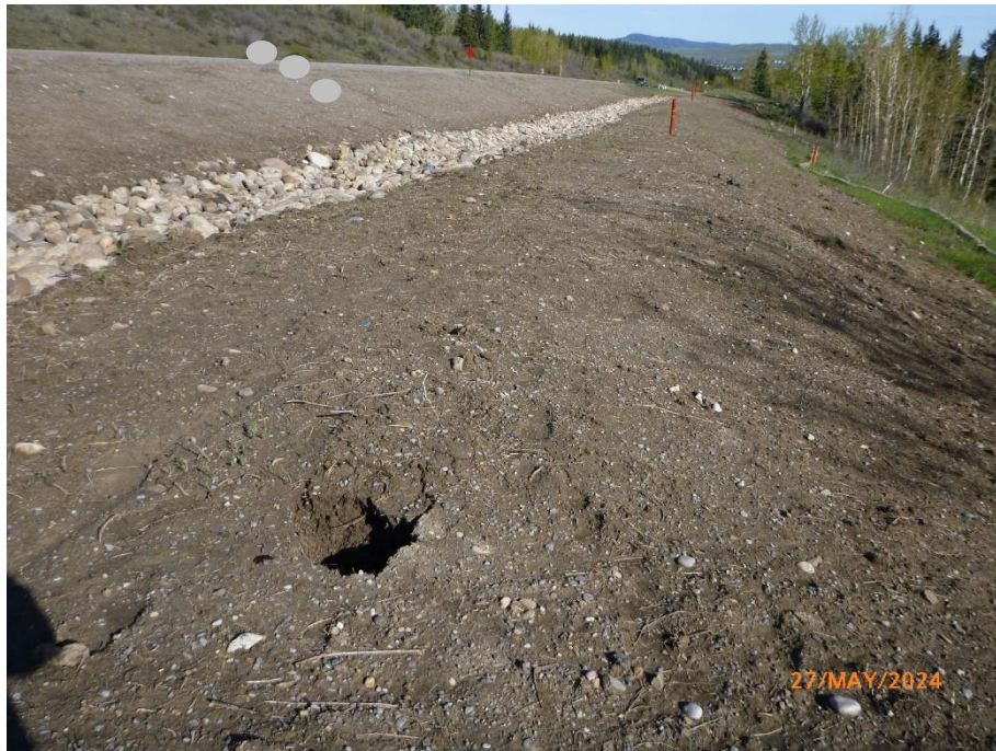
Photo 4 Pile wall alignment. Some voids forming in the pile flanges due to backfill settlement. Photo taken facing north on May 27, 2024.
