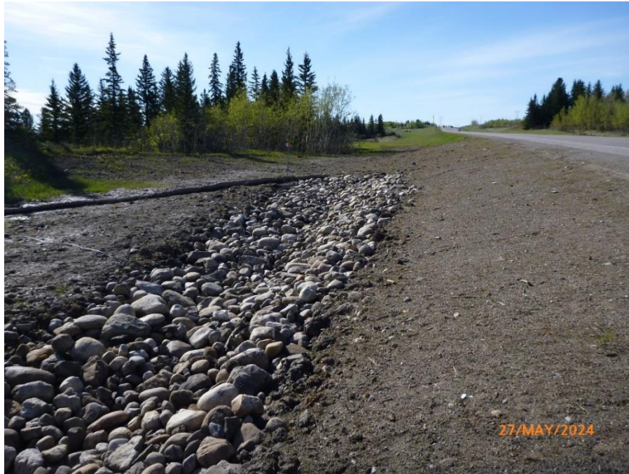
Photo 2 North end of the project area with the ditch reinstated with riprap. Pile wall installed downslope of ditch. Photo was taken facing northwest on May 27, 2024.
