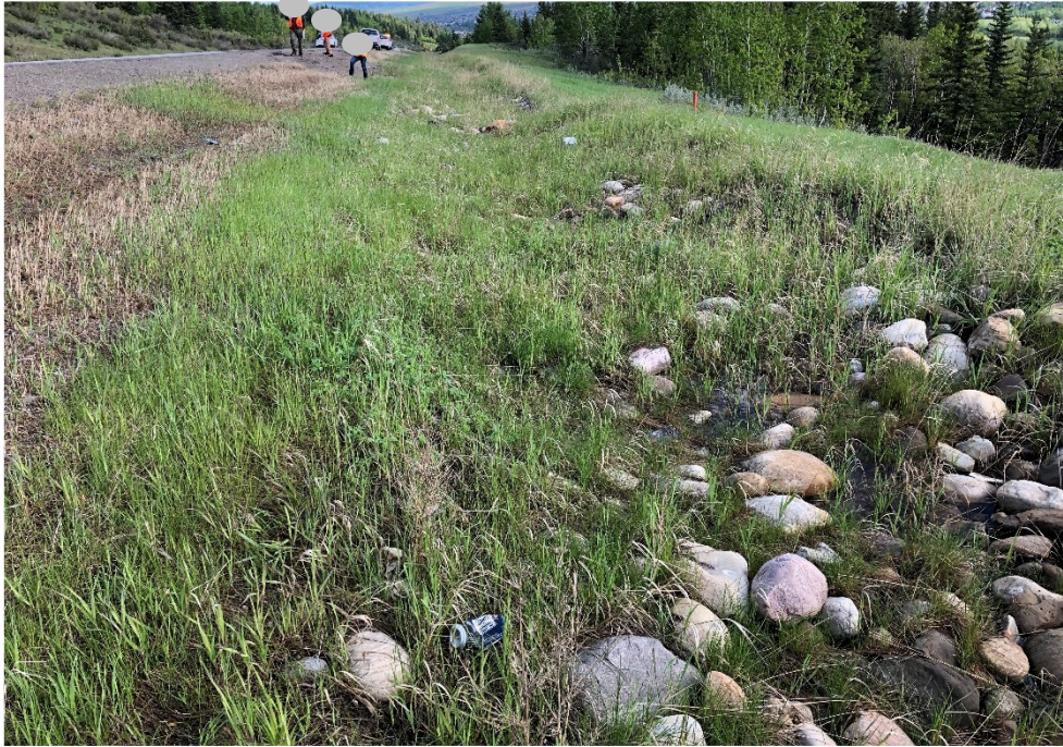
Photo 4 Tension cracking near fence line due to midslope movement (minor scarp). Photo taken facing north on June 8, 2020.
