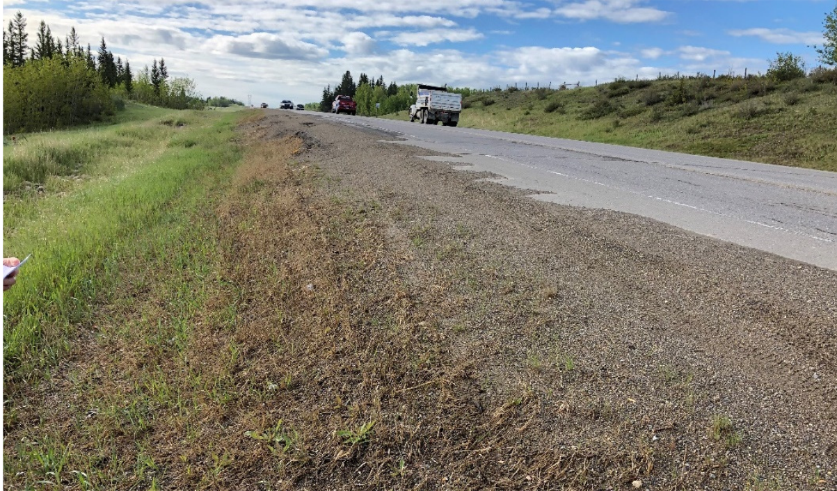
Photo 2 Cracking and settlement on the highway shoulder approximately 3 m into the lane (red arrow). Photo taken facing northwest on June 8, 2020.
