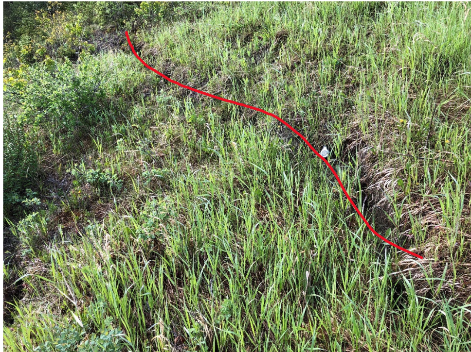
Photo 4 Tension cracking near fence line due to midslope movement (minor scarp). Photo taken facing north on June 8, 2020.
