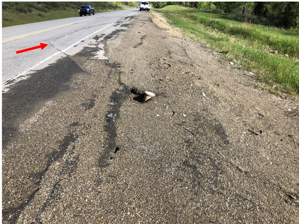
Photo 2 Cracking and settlement on the highway shoulder approximately 3 m into the lane (red arrow). Photo taken facing northwest on June 8, 2020.
