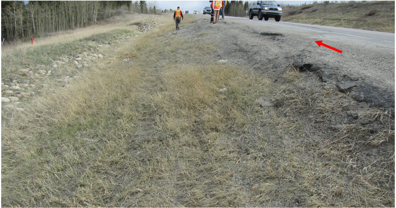
Photo 2 Cracking and settlement on the highway shoulder. Photo taken facing northwest on May 7, 2019.
