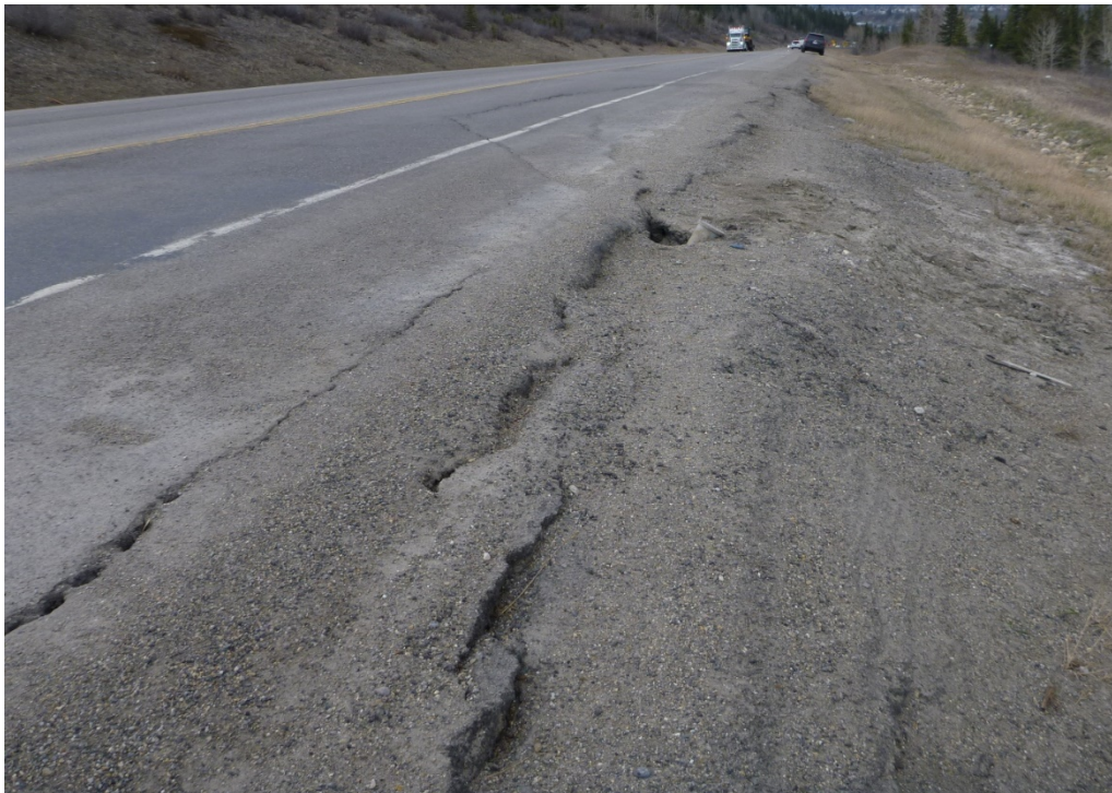
Photo 2 Cracking and settlement on the highway shoulder. Photo taken facing northwest on May 7, 2019.
