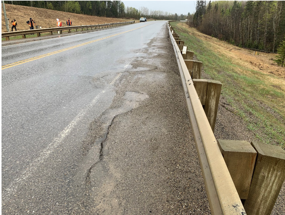
Photo 2 Cracking at the east extent of the slide on the highway. Photo taken facing west on May 9, 2023.
