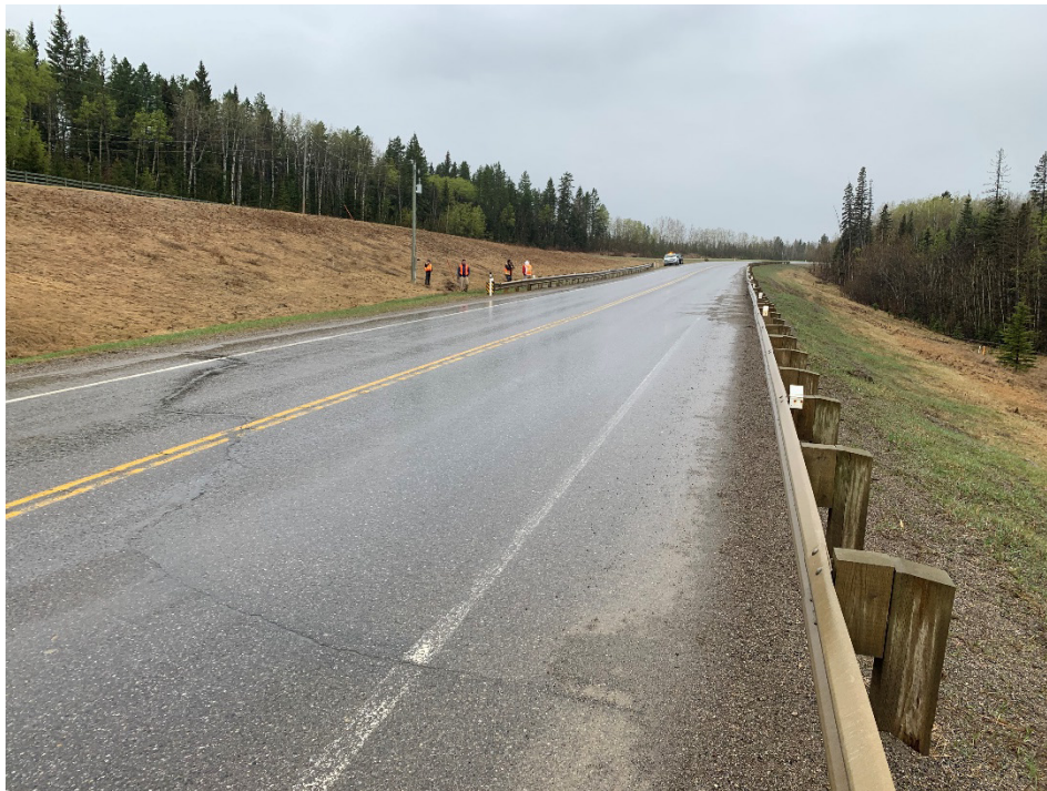
Photo 2 Cracking at the east extent of the slide on the highway. Photo taken facing west on May 9, 2023.
