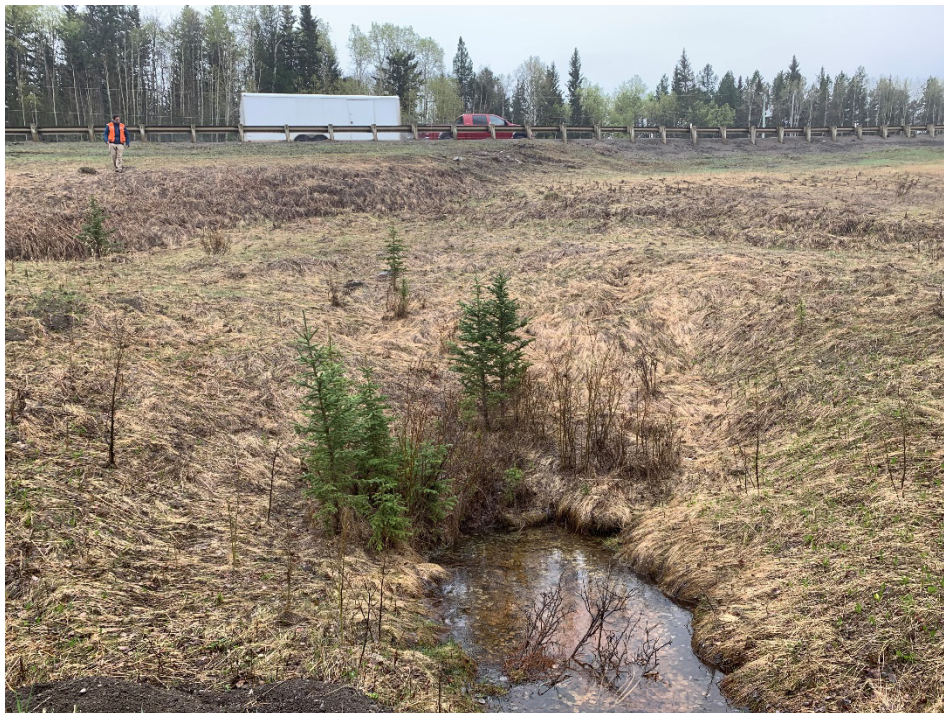
Photo 6 Ponded water at the toe of the slope. Photo taken facing south on May 9, 2023.
