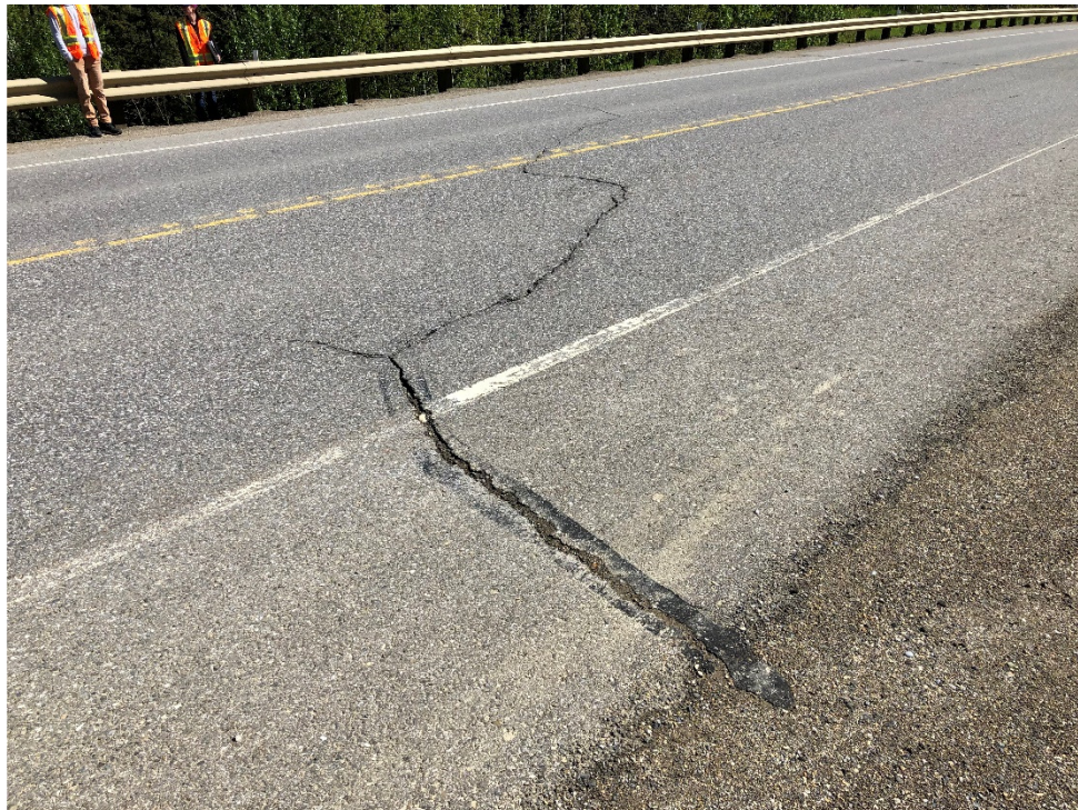
Photo 4 Pavement cracking has extended northwards when compared to 2019 observations. Photo taken from south side of highway facing northeast on June 8, 2020.
