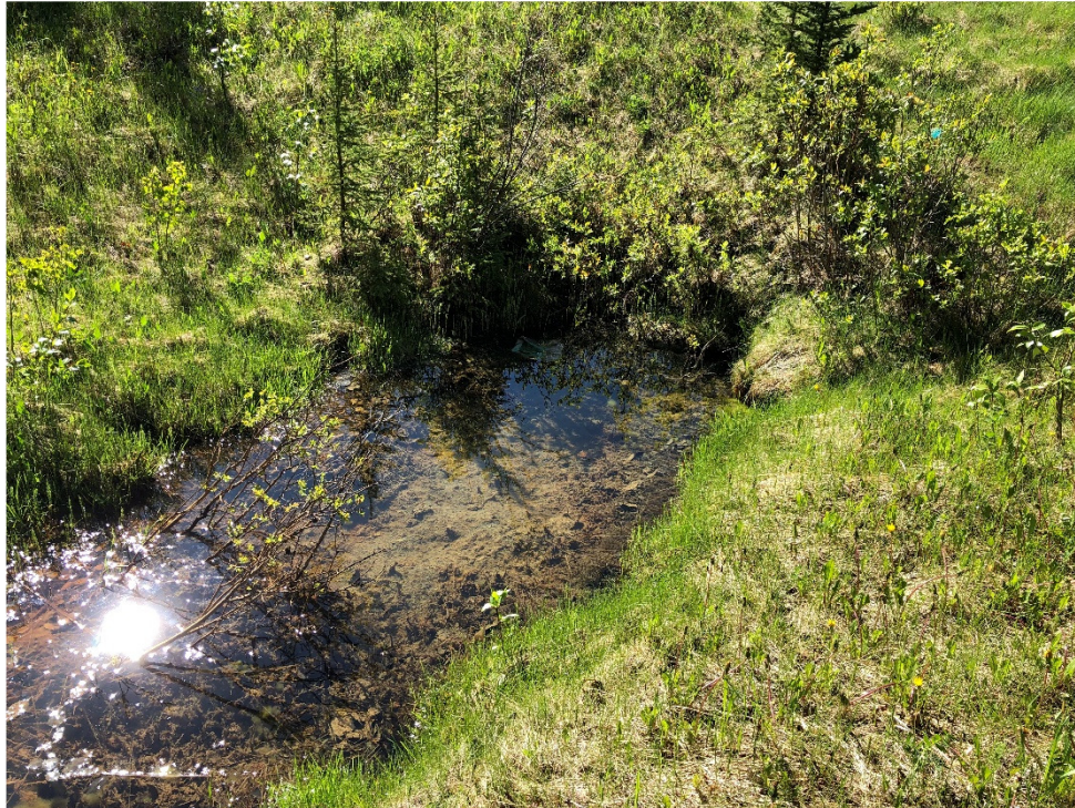
Photo 5 Ponded water at the toe of the slope facing southeast. June 8, 2020.
