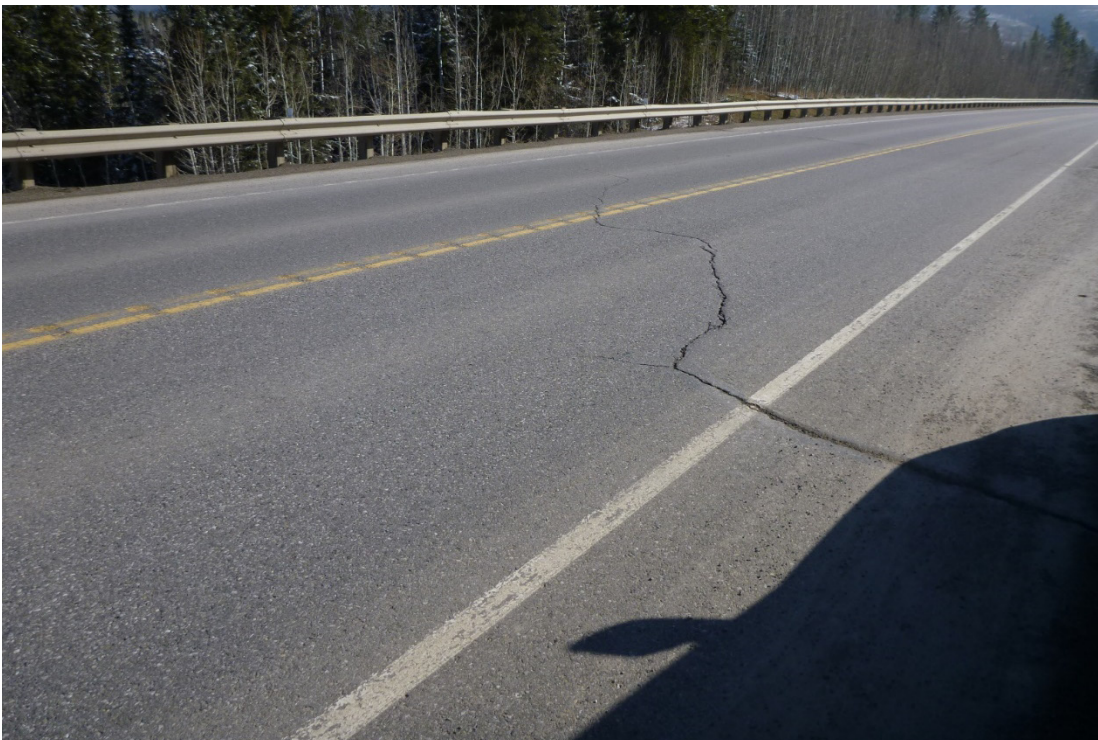
Photo 4 Pavement cracking. Photo taken from south side of highway facing northeast on May 6, 2019.
