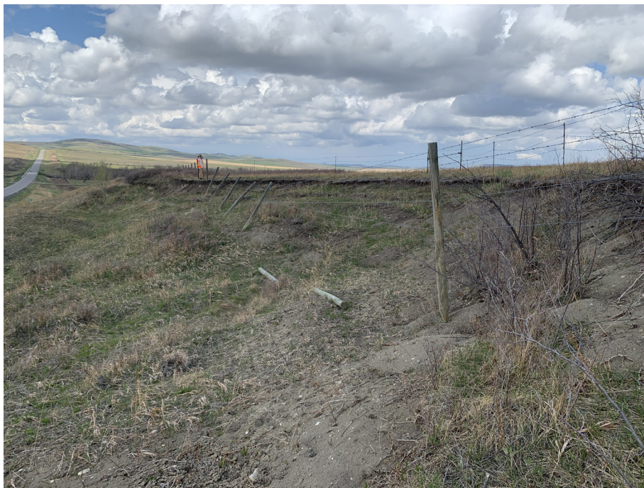
Photo 2 Approximately 36 m length of undermined fence line at crest of slope. Photo taken facing north on May 9, 2023.
