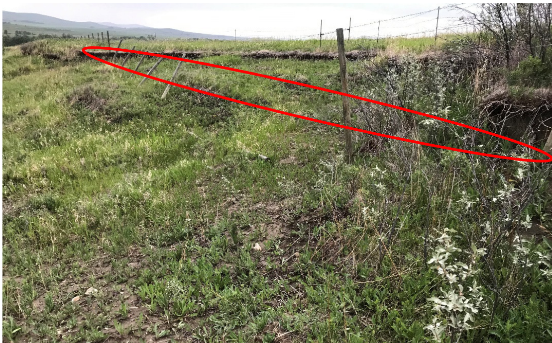
Photo 2 Approximately 36 m length of undermined fence line at crest of slope. Photo taken facing northeast on July 5, 2021.
