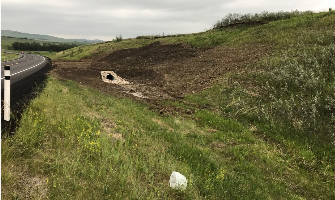
Photo 4 Culvert installation and ditch regrading on east side of the highway completed during 2021 paving activities. Photo taken facing south on July 5, 2021.
