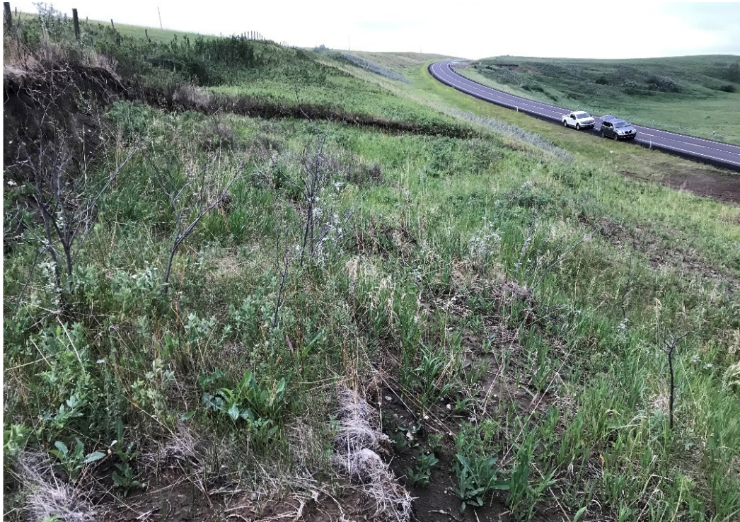
Photo 2 Approximately 36 m length of undermined fence line at crest of slope. Photo taken facing northeast on July 5, 2021.
