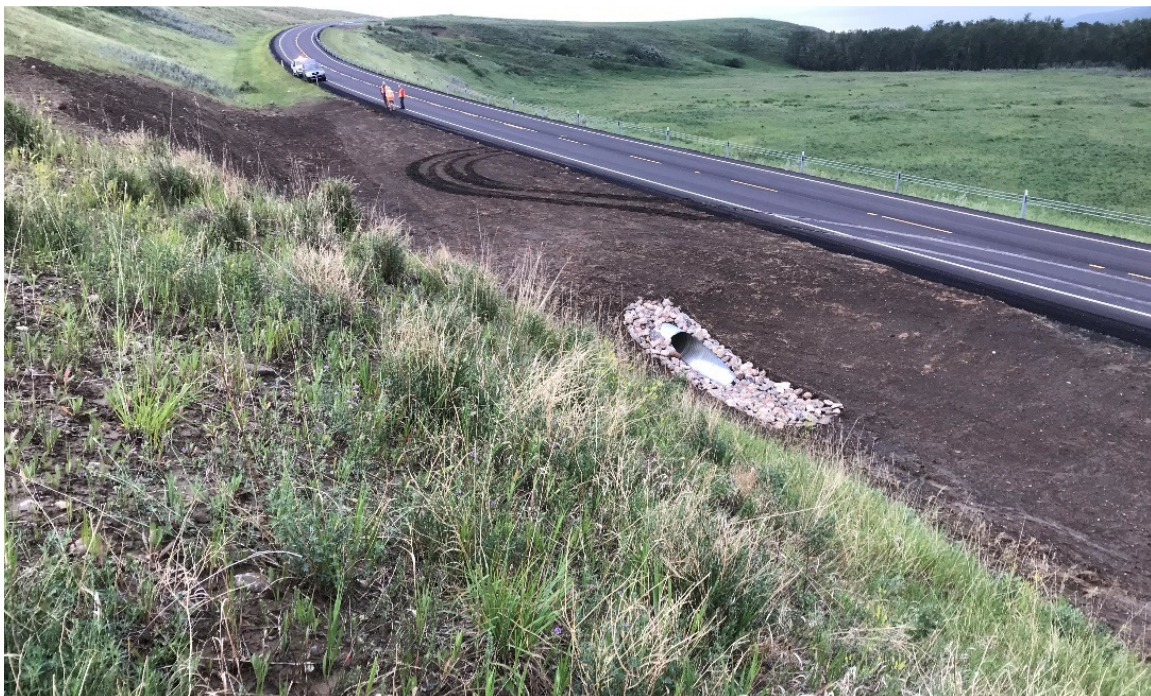
Photo 4 Culvert installation and ditch regrading on east side of the highway completed during 2021 paving activities. Photo taken facing south on July 5, 2021.
