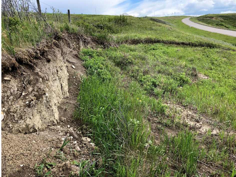
Photo 2 Approximately 36 m length of undermined fence line at crest of slope. Photo taken facing northeast on June 8, 2020.
