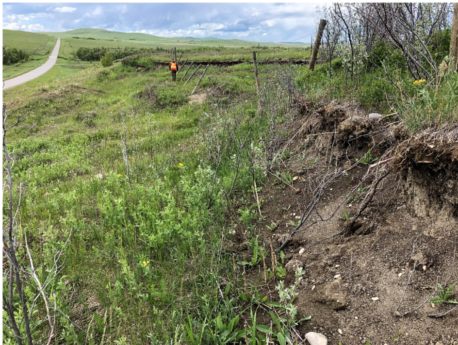
Photo 2 Approximately 36 m length of undermined fence line at crest of slope. Photo taken facing northeast on June 8, 2020.
