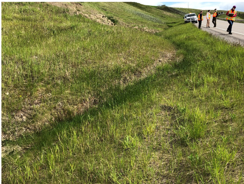
Photo 4 Toe rolls partially blocking the ditch. Photo taken from east side of highway facing southeast on June 8, 2020.
