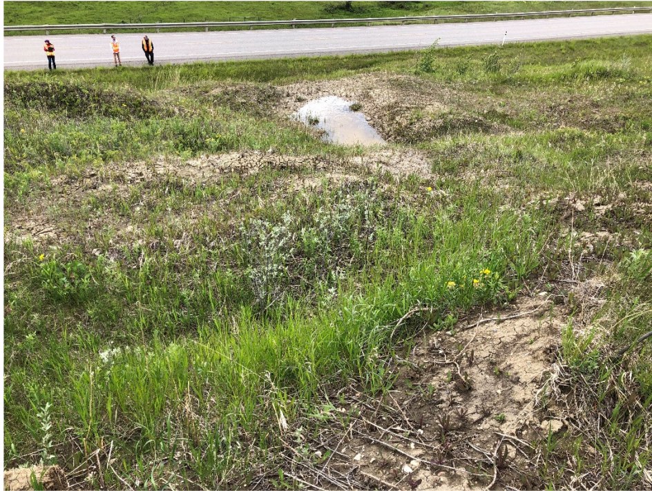
Photo 4 Toe rolls partially blocking the ditch. Photo taken from east side of highway facing southeast on June 8, 2020.
